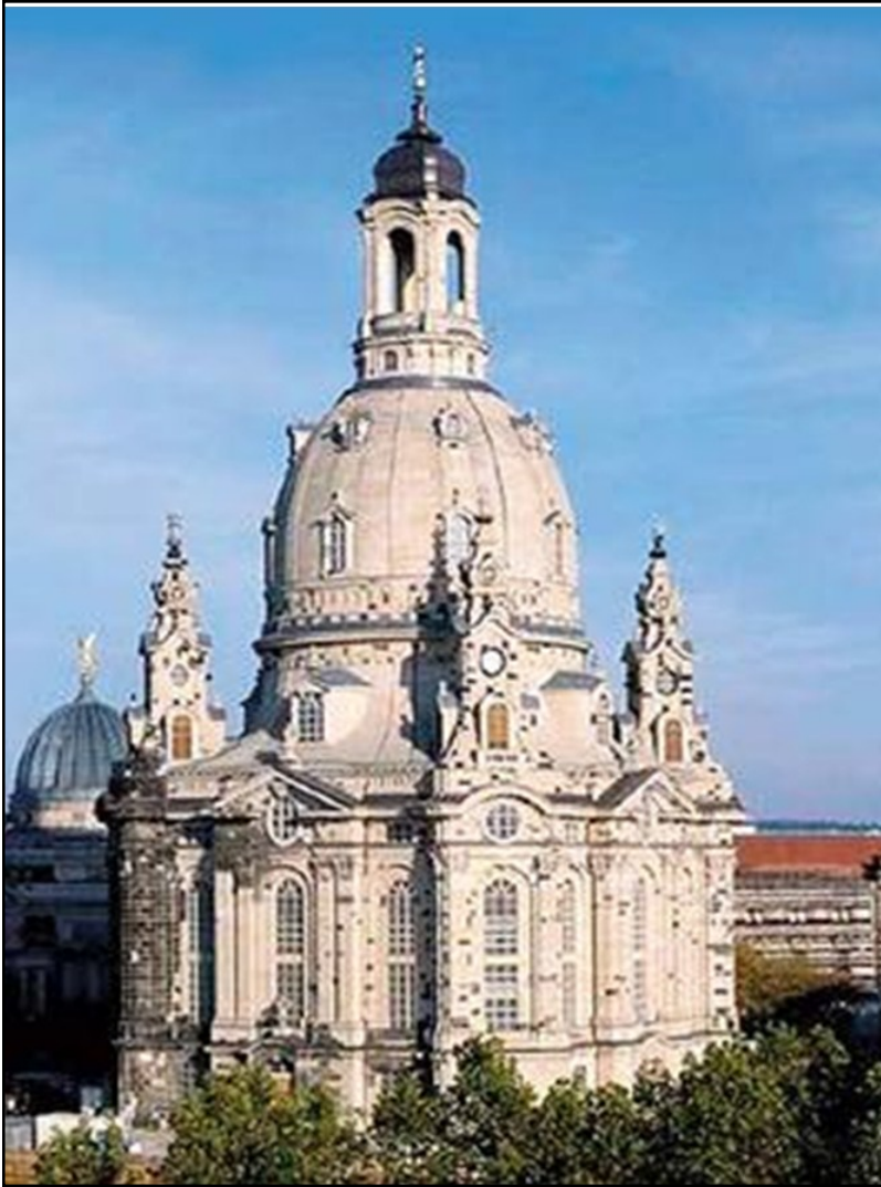
Figure 2.9: The reconstructed Frauenkirche with darker, original stones visible in the lower, left hand corner of the structure. Image from Frauenkirche website.
