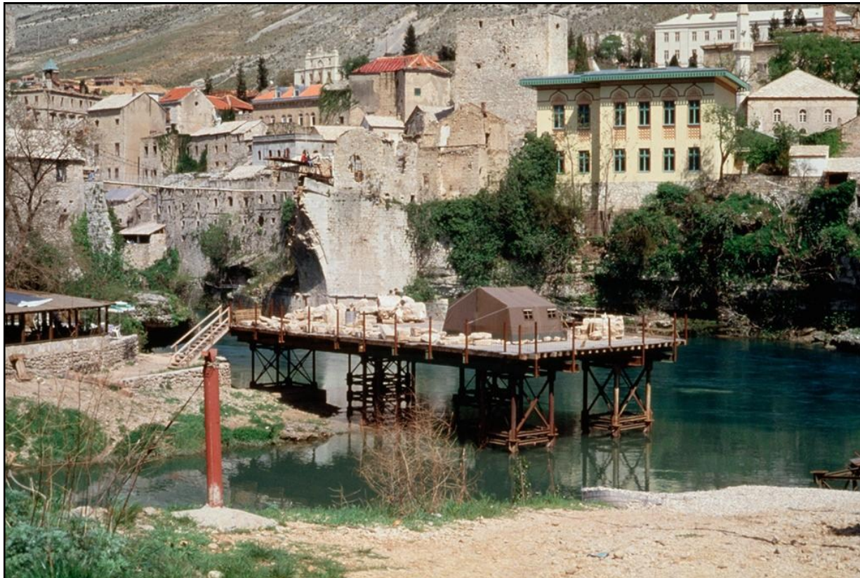
Figure 13: Photograph of the staging for the salvage and reconstruction of Stari Most in 1998. Photography by Jon Calame.
