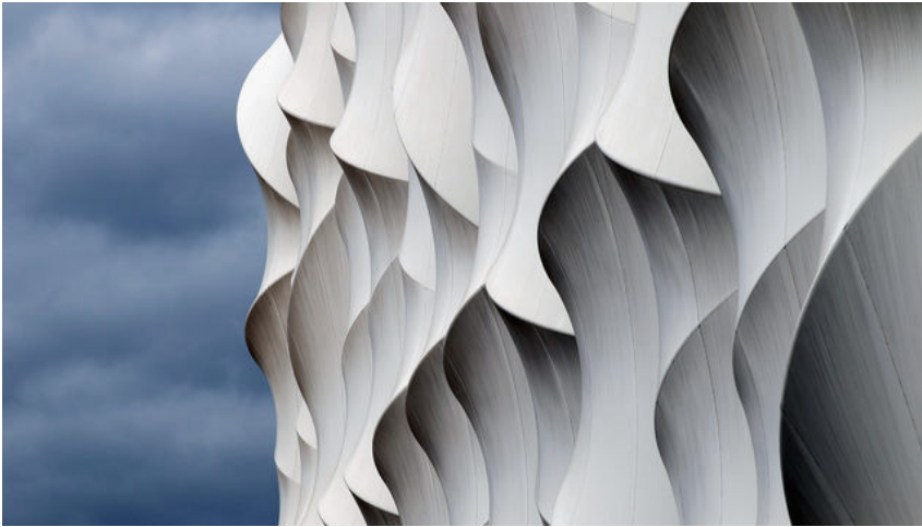
Figure 6: Undulating Facade of the London Basketball Arena
