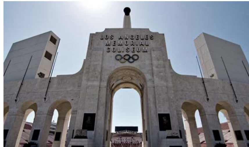
Figure 4: Los Angeles Memorial Coliseum in Los Angeles, California
