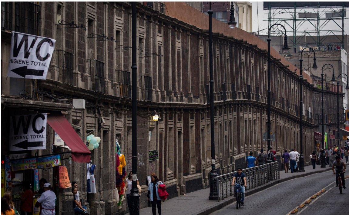
Figure 43. Street in Mexico City demonstrating uneven settlement due to overdrawn aquifer.
