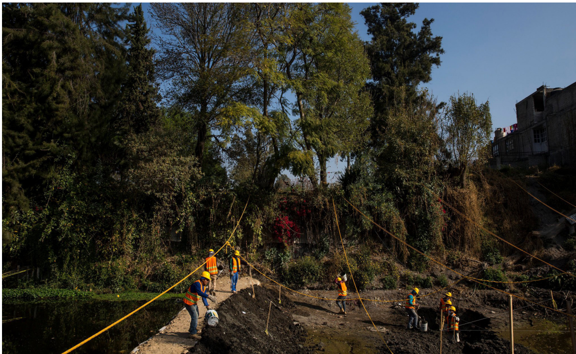
Figure 47. Fixing the fissure hole.
