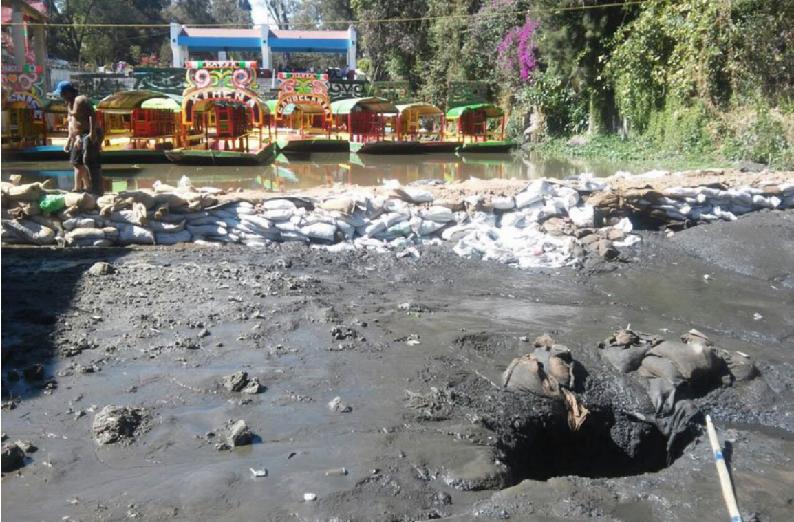
Figure 48. Fissure at the Xochimilco Canals.
