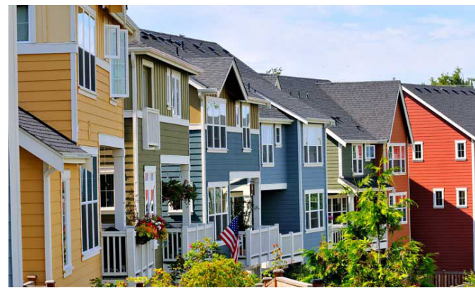
Figure 5.4 High Point typical streetscape
