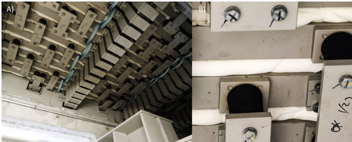
Figure 2.10: Underside of the MEJ with viscoelastic foam strips stuffed into the gaps. (A) Overview photograph. (B) Detailed view.
