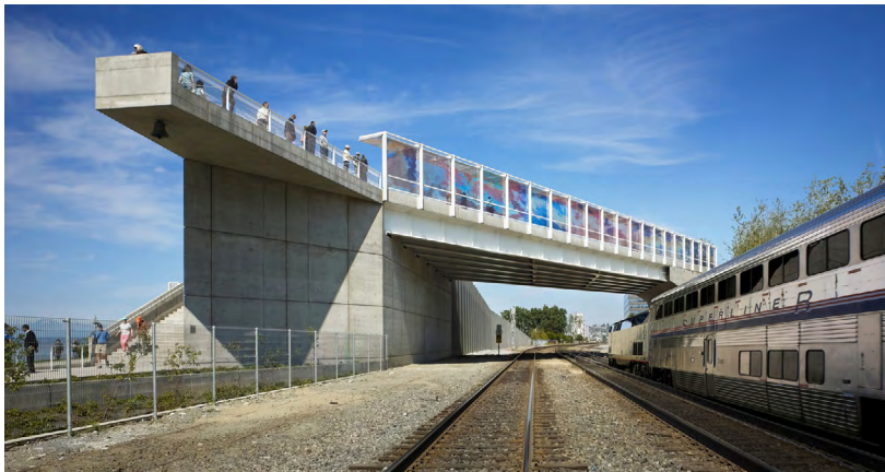
Figure 89: Walkway Over the Rails
