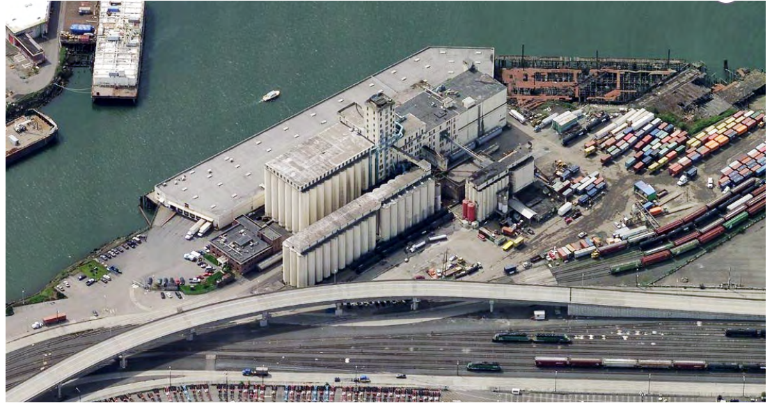
Figure 14: The mill's current condition (looking west)
