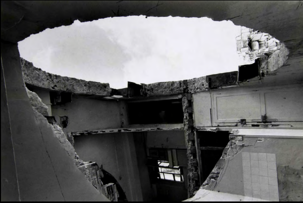
Figure 58: Building cut by Gordon Matta Clark
