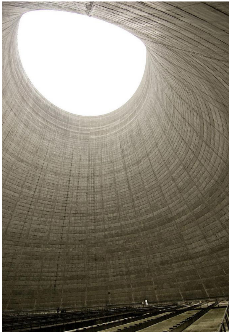
Fig. 29 Inside Satsop cooling tower
