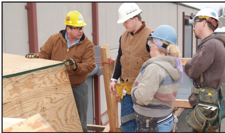
Instructor Dan Voight (left) explains the basics of bridge building to apprentices Jim Bender, Raeleen Ross and Reid Stephens. The Willamette Carpenters Training Center has a section of a mock bridge constructed by apprentices on the back lot of its new facility in Northeast Portland.
