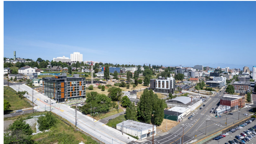
Main Expansion Area - heading up the Hill towards Tacoma Ave S
