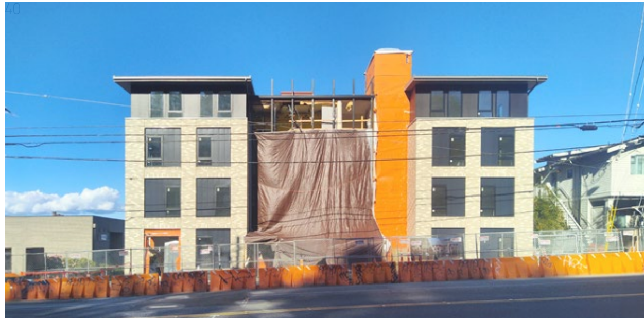
Figure 11: Image of 2514 Dexter Ave N under construction in spring of 2023.
