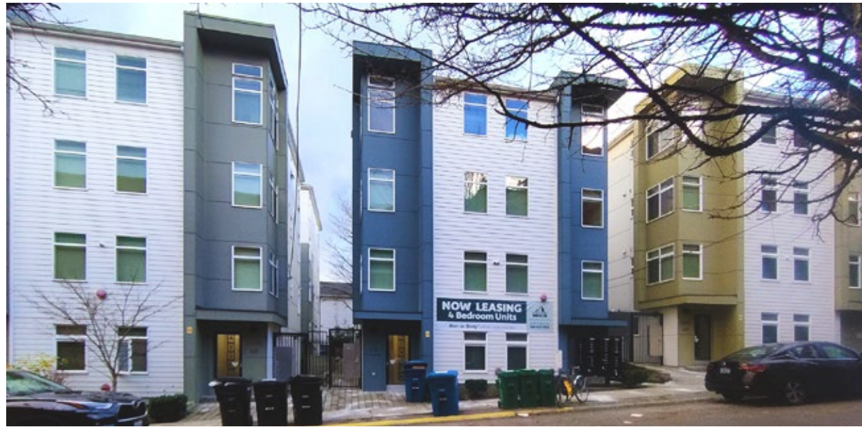
Figure 40: All three of these buildings, located in the University District, share identical floor plans favoring roommates rather than families.
