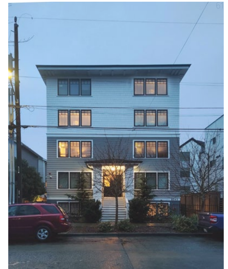
Figure 53: Photo of 8543 Midvale Ave N taken in early 2024.
