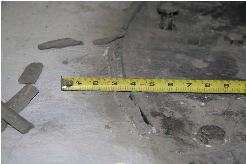
Figure 6.35. North Side of Ring Flange – After Test (PTB_9_2_0_P)
