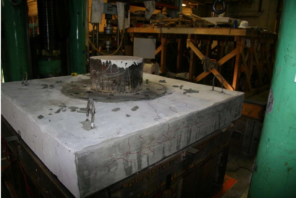
Figure 6.39. Cracking East Face – Load Removed (PTB_9_2_0_P)
