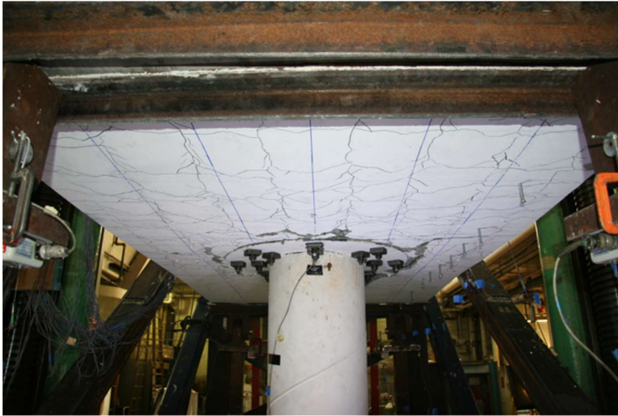
Figure 4.47. Damage on North Side of Bottom Face– 5.61% Drift (PTB_9_2_0_6)
