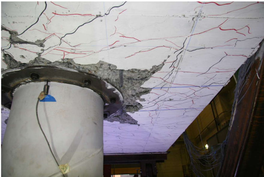
Figure 4.23. Crushing on South Side of Bottom Face – 5.63% Drift (PTB_4.5_1_0_6)
