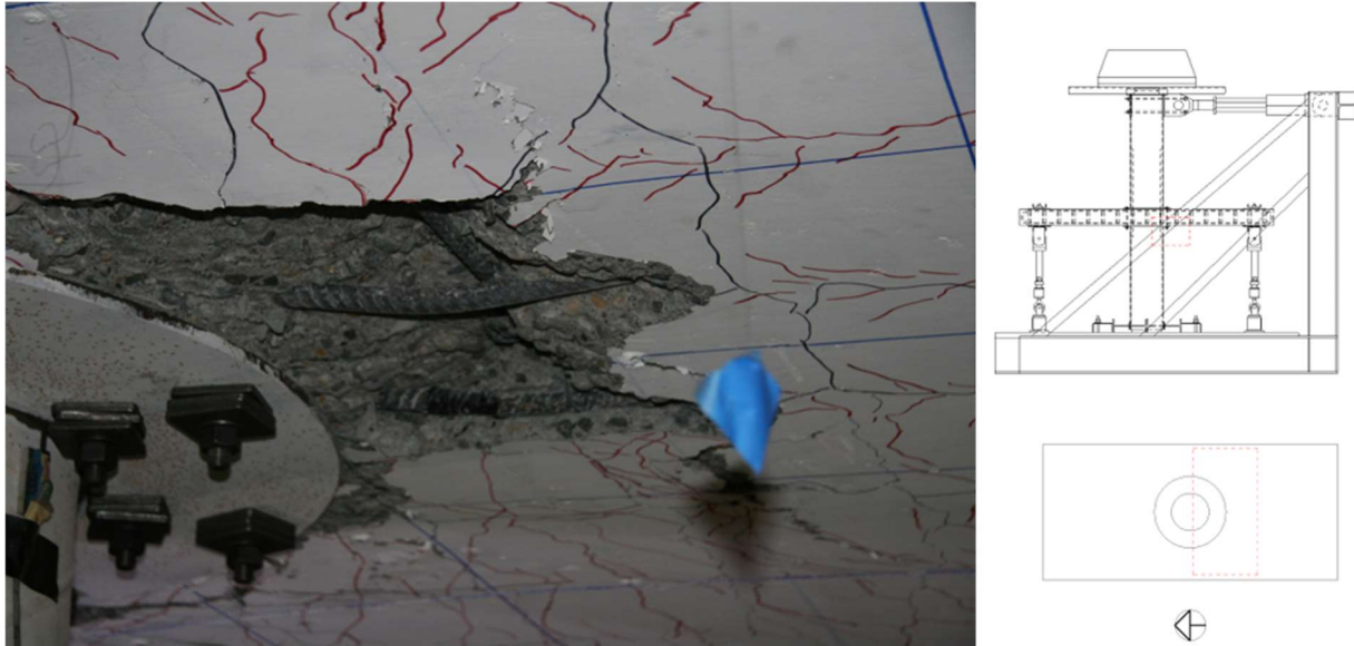
Figure 4.5. Example of Bar Buckling
