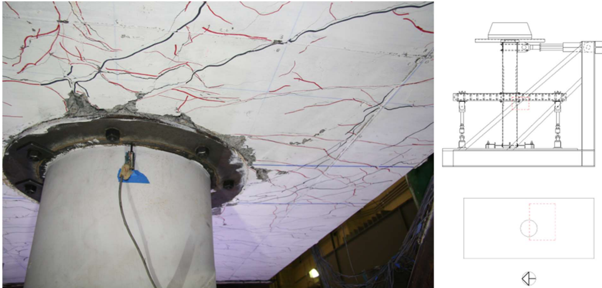
Figure 4.4. Example of Core Concrete Crushing
