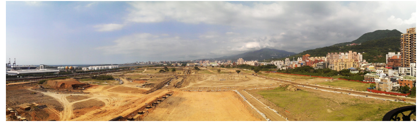
Fig 5.4 Looking east across the site
