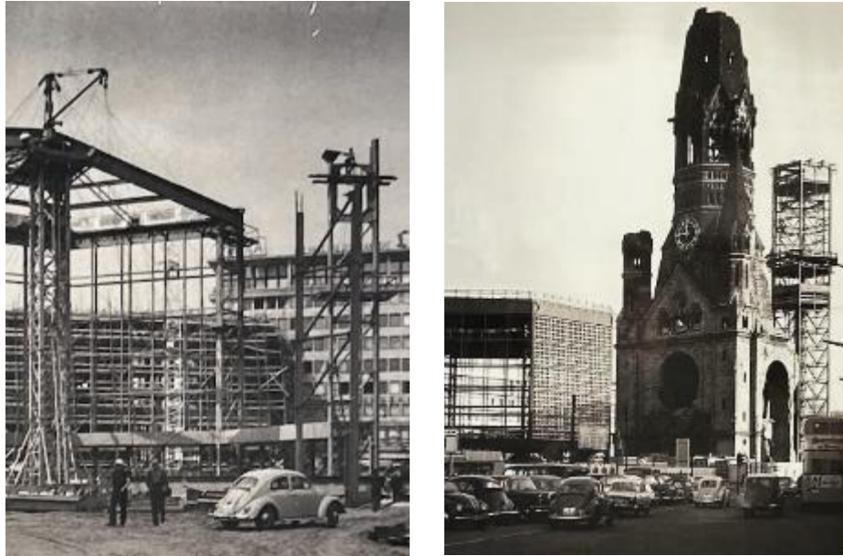
Figure 26. New bell tower and nave under construction. Circa 1959-1962 © KWG Archives
