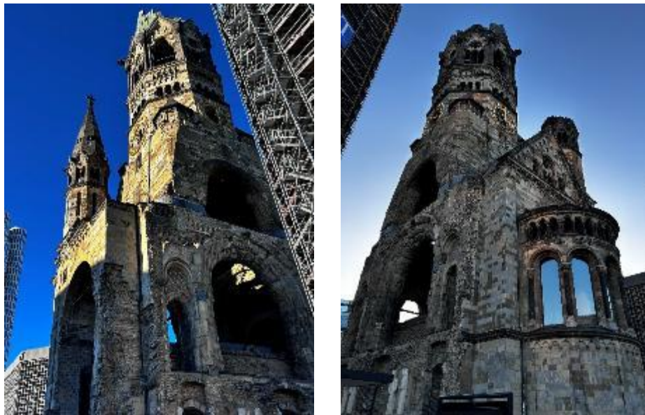
Figure 30. External views of the old tower © Photo by Author
