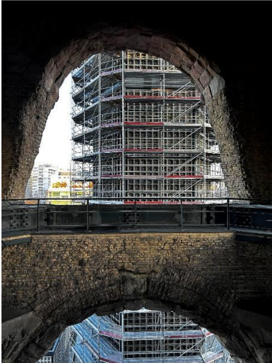
Figure 34. View of the new bell tower from the old tower © Photo by Author
