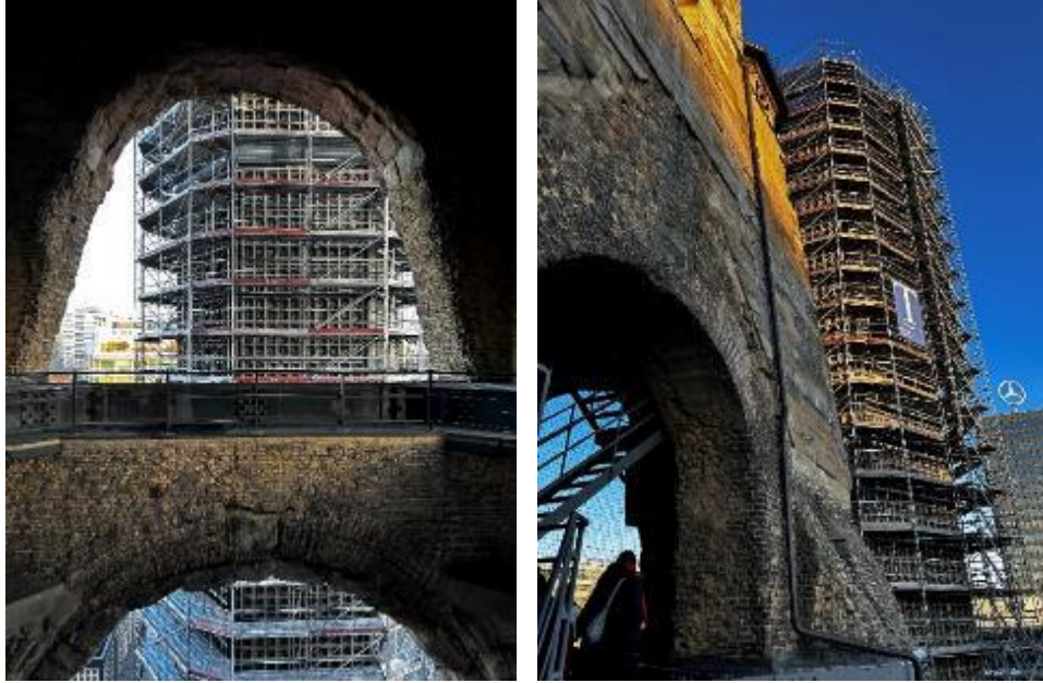
Figure 10. Scaffolding around the new Bell Tower, from the old tower © Photos by Author
