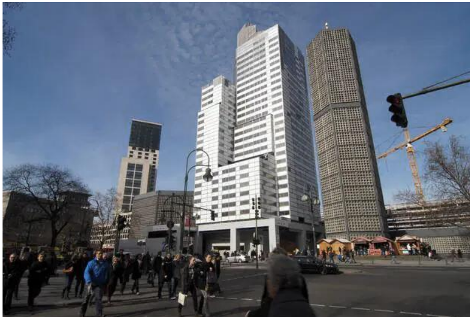
Figure 8. Scaffolding resembling an office building ©imago
