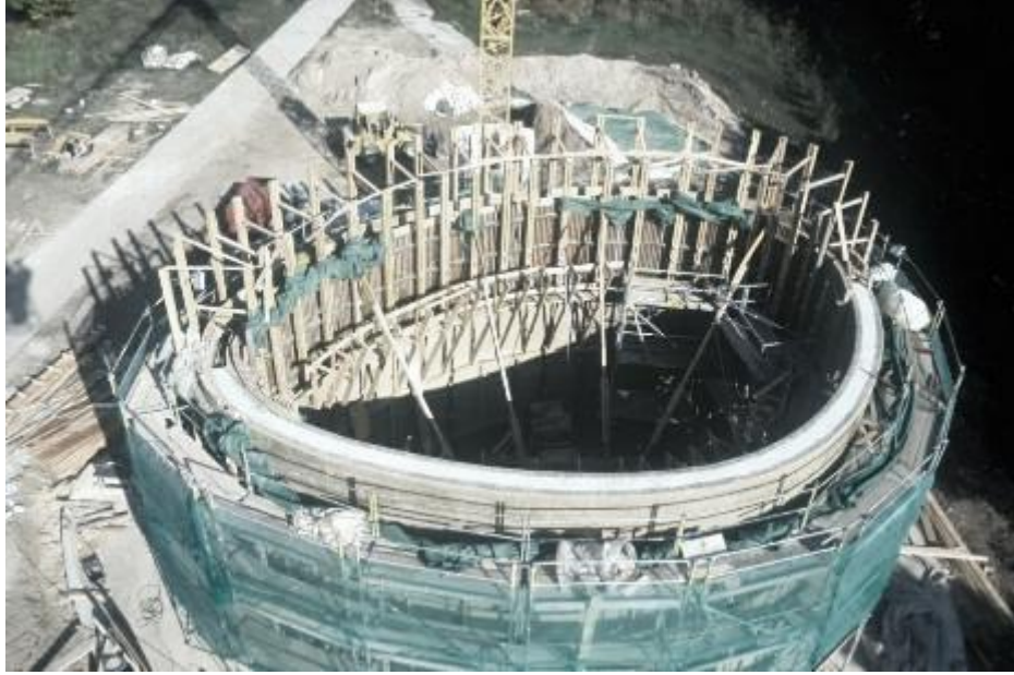
Figure 52. Chapel of Reconciliation under construction © ZRS Architects Engineers
