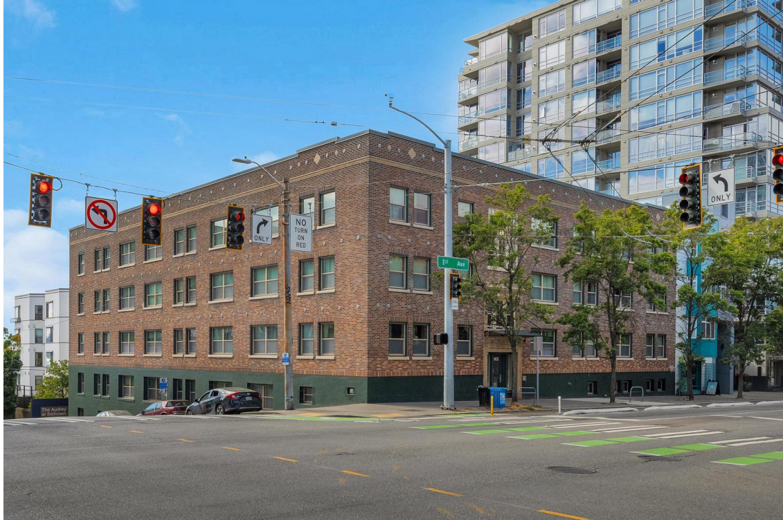
Figure 2. The Bremer Apartments. Source: Historic Seattle 2022.
