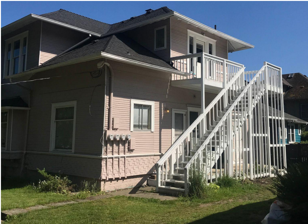
Figure 26. The front (above) and back (below) of the triplex at 4533 Eastern Ave. Photos by Charlotte Hevly.
