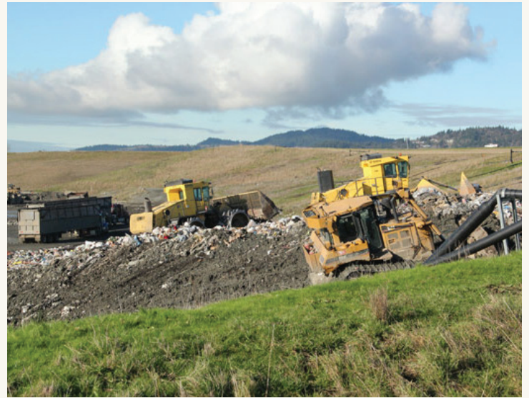
Fig. 42 Waste at the CHRLF is pushed into cells. Photo: King County. Photo: King County
