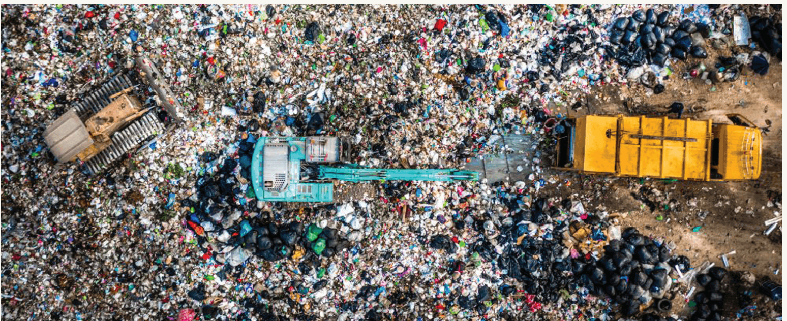
Fig. 47 Aerial photograph of landfill being mined. Photo: Eric Lawson, waste360.com
