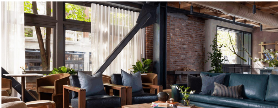
Fig 23: A typical steel frame used for seismically retrofitting a URM building. Source: https://millerhull.com/project/populus-seattle/
