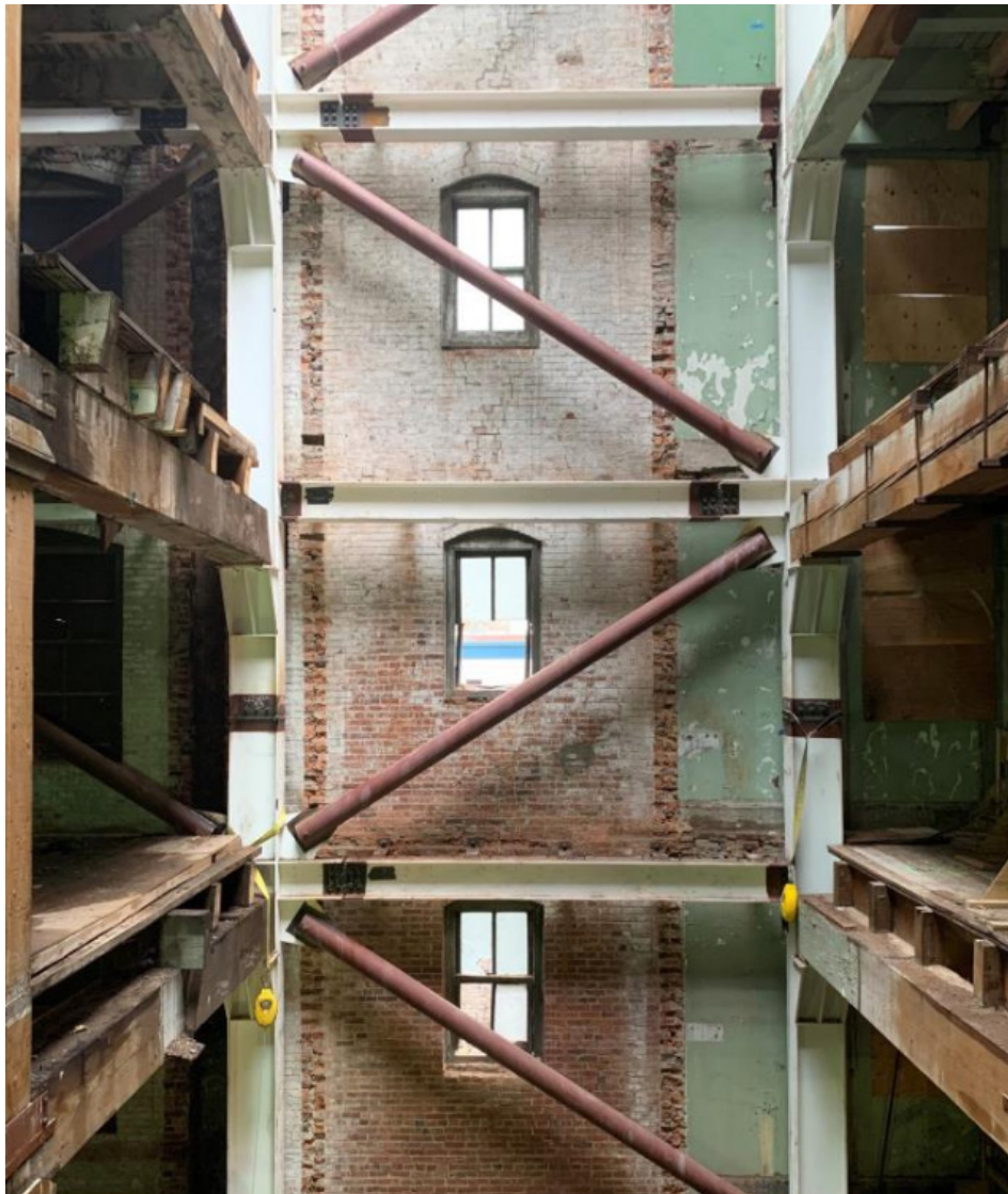
Fig 28: Photo depicting extensive selective demolition for integration of steel bracing in a URM building seismic retrofit. Source: Swenson Say Faget
