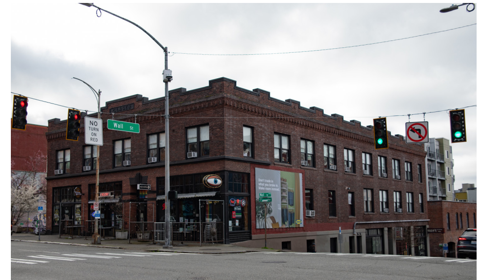
Fig 17: Photo of a commercial/residential mixed use URM building. Source: Photo by author
