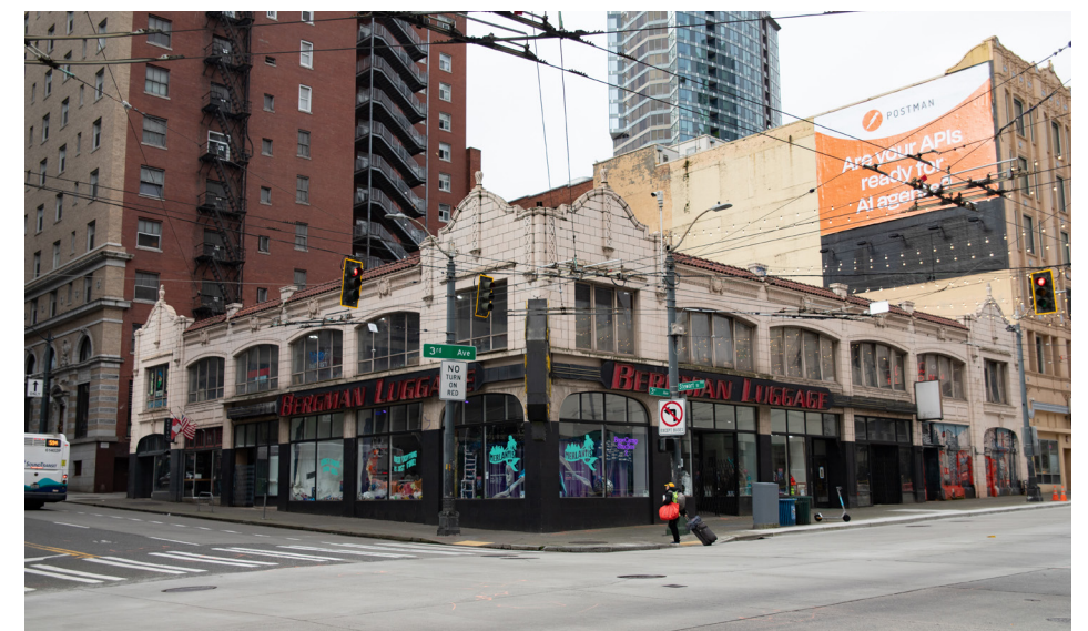
Fig 19: Photo of a commercial mixed-use URM building. Source: Photo by author
