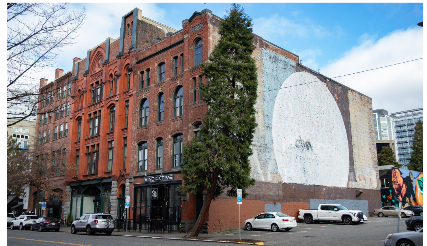
Fig 68: The west and south facade of the Barnes Building. Source: Photo by author
