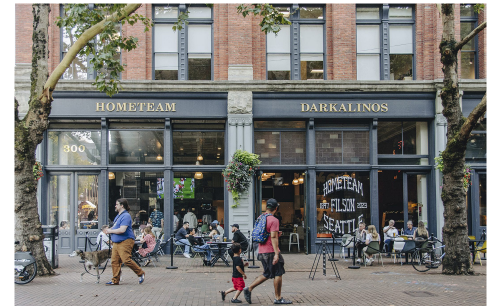
Fig 3: Typical URM building storefront.
