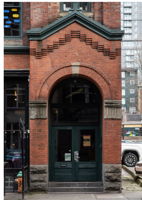
Barnes building entry details
