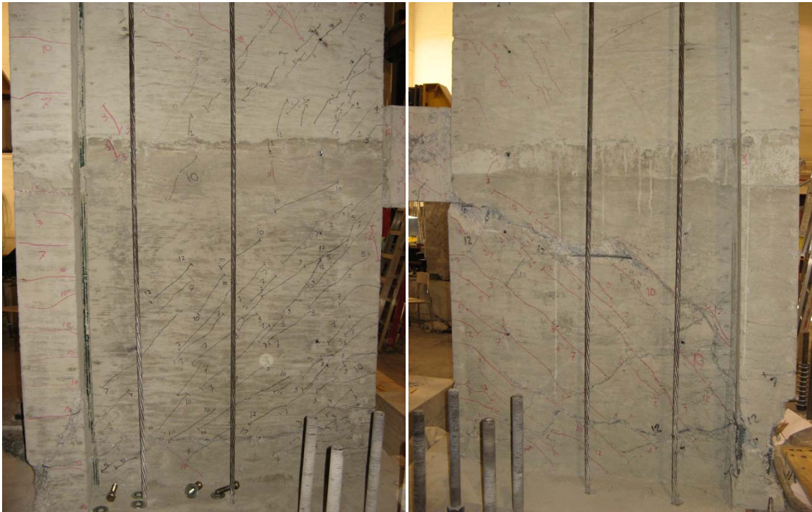
(b) Base of CW2 (rear view)
