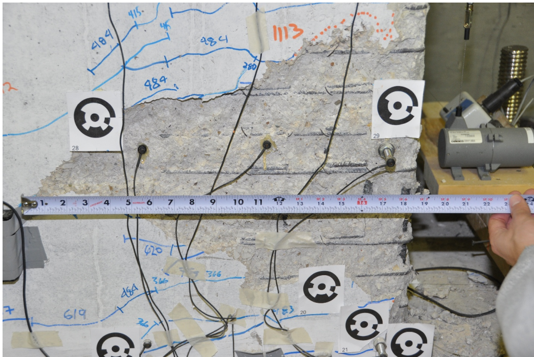
Figure 4.32: Spalling of EWP at 2.20% (2.25% D.C. (A), Step 954)
