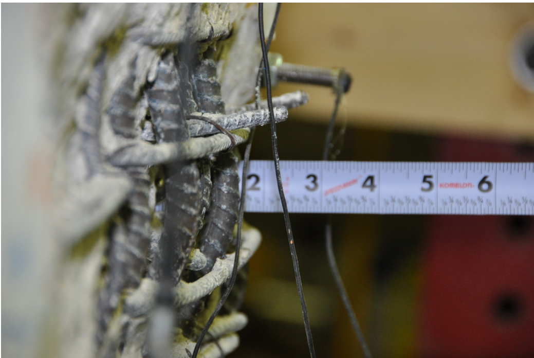
Figure 4.34: Buckled rebar on south facing side of EWP at E+ peak
