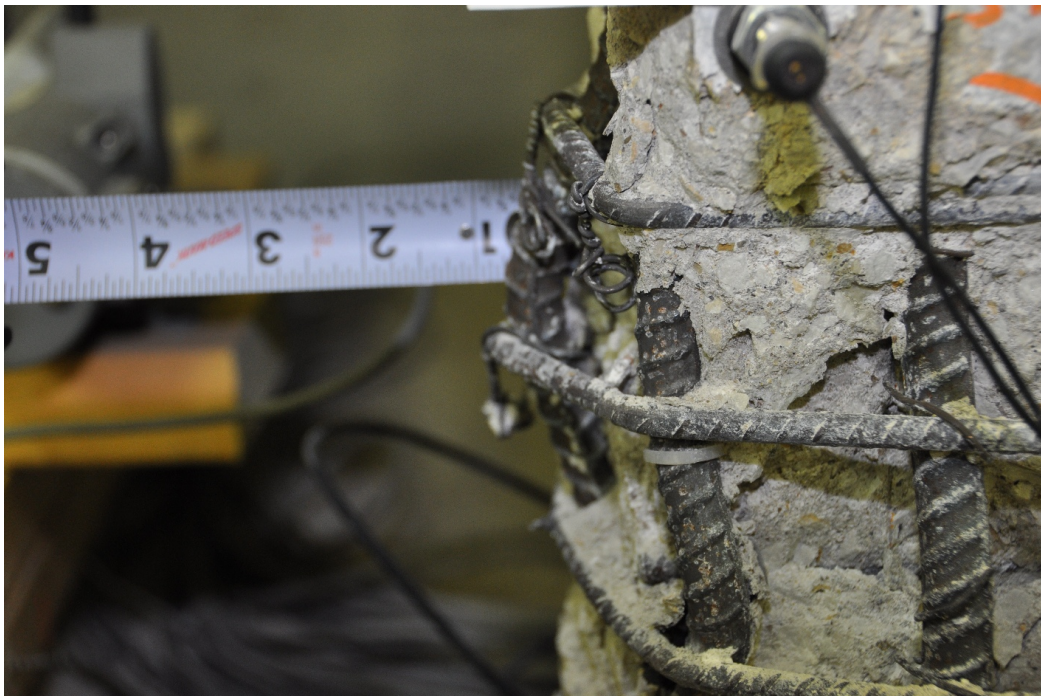
Figure 4.40: Close-up of WWP buckled rebar at W- peak (2.25% D.C. (A), Step 1003)
