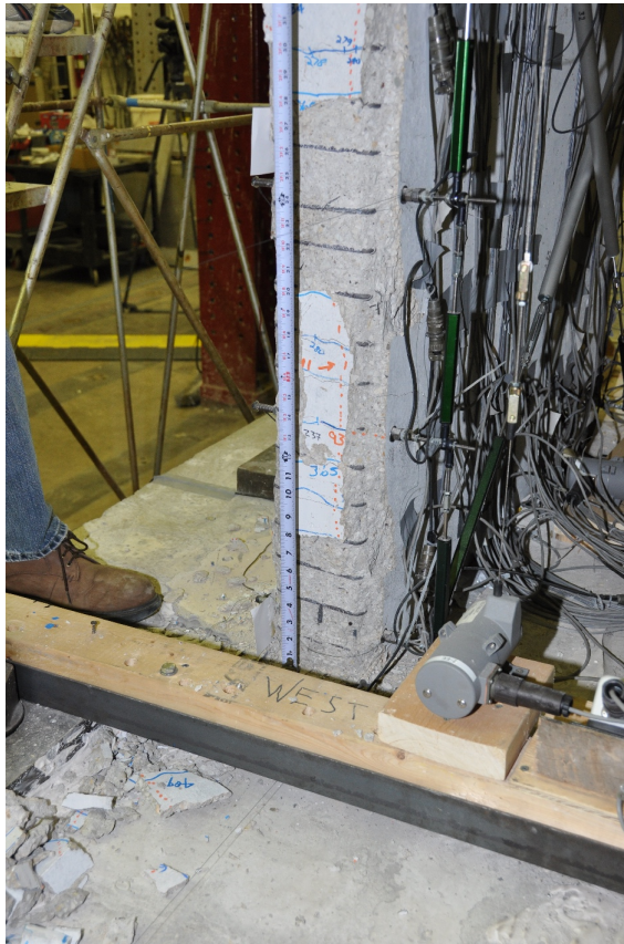
Figure 4.26: Spalling of EWP at the end of the 1.50% drift level, top of spalling shown 28 inches above wall base
