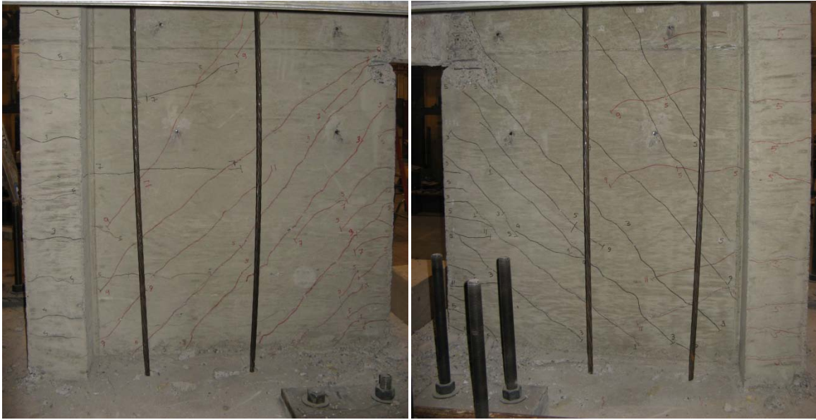
(a) Base of CW1 (rear view)
