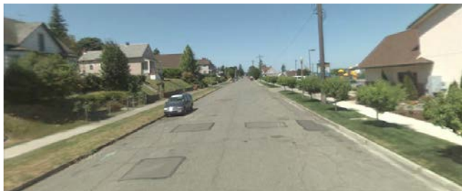
Figure 9: South G Street
