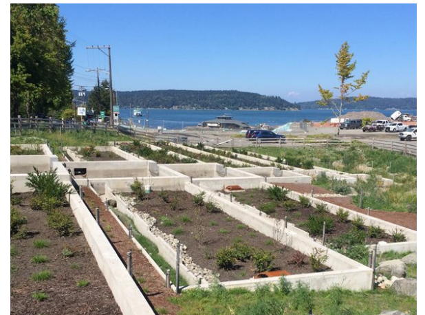
3 - Stormwater Filtration Terraces
