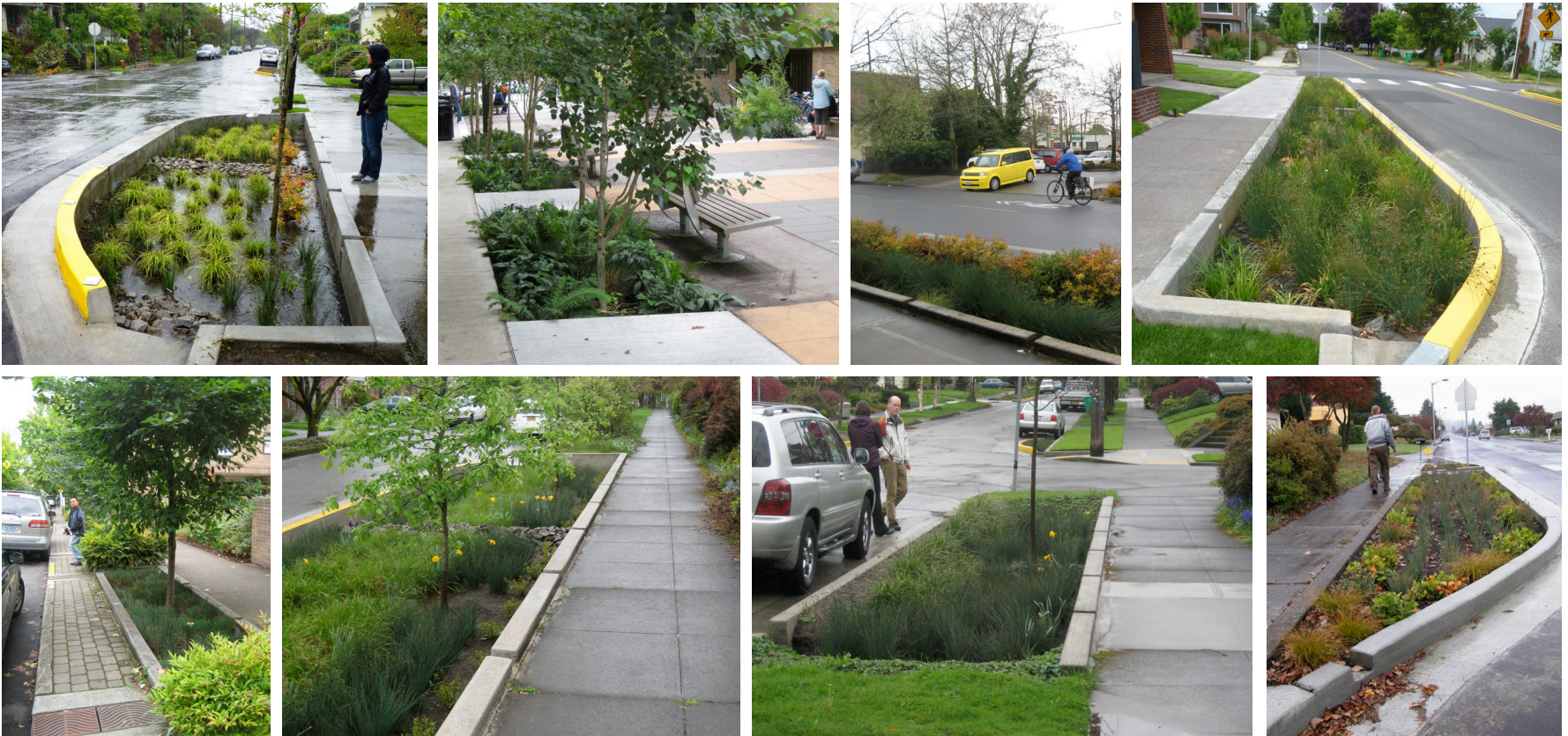
Figure 24: Vertical Side Walls in Residential and High Foot Traffic Settings
