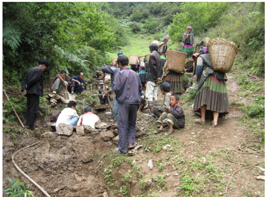
Figure 17: Villagers Participating in New Reservoir Construction
