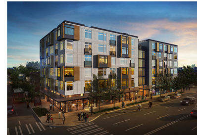
The Central (Under Construction) 2203 E Union St 2015
