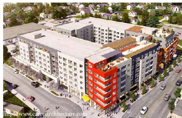
Othello Station North
