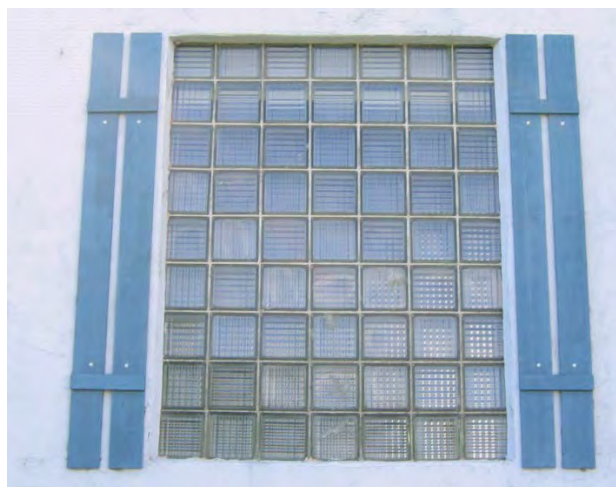
Figure 7.16: Manson #796 in Chelan County (Detail of windows)
