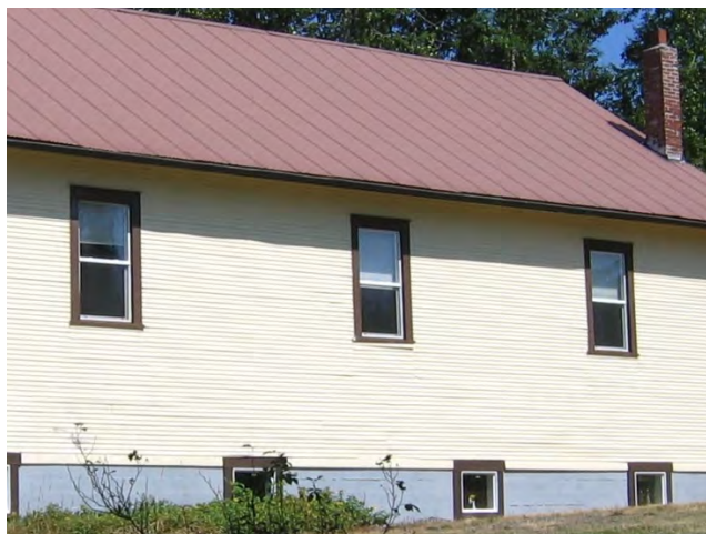
Figure 7.15: Rome #226 in Whatcom County (Detail of windows)
