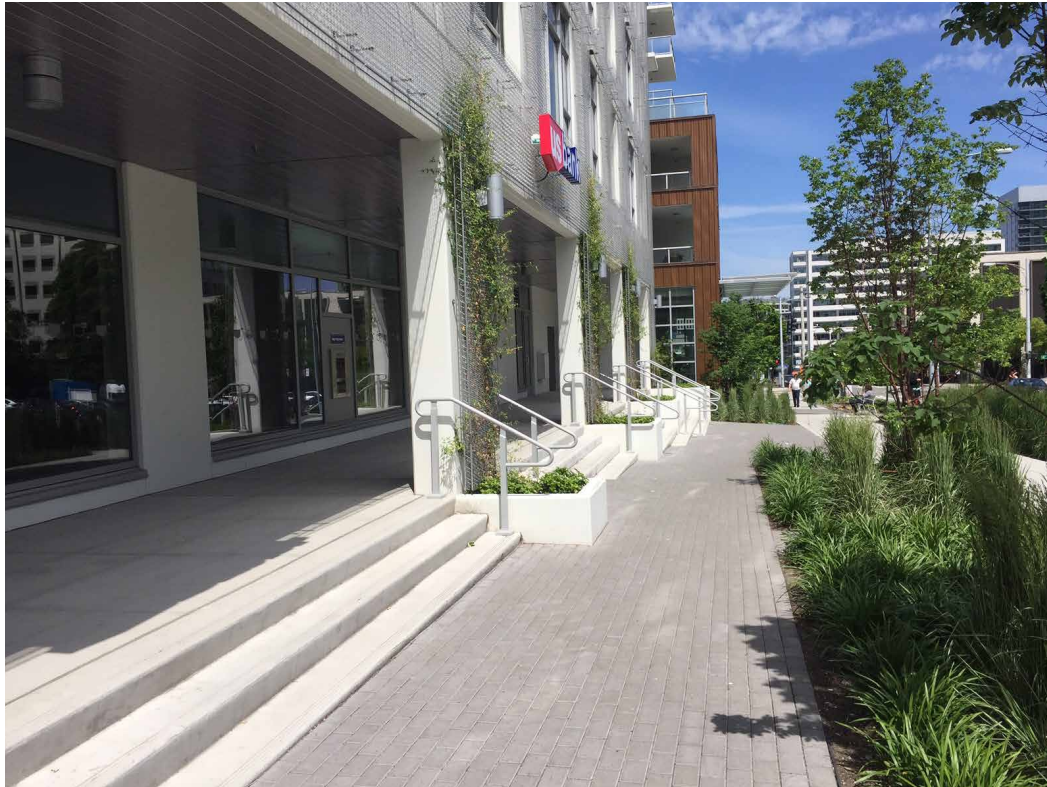
Figure 46: Covered walkway on north side of Bell Street.
