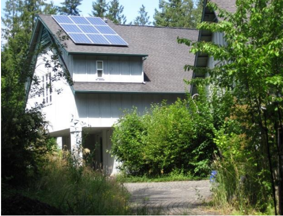
Photo 2.3: Northwest Stream Center (Hanson 2011)
