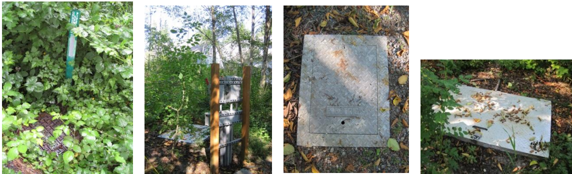
Photos 3.59-3.62: (L to R) Some of the site utilities that would need to be located and marked are near the gravel path in the northwest corner by the trout stream in sectors 161 and 183 (photos Hanson 2011).
