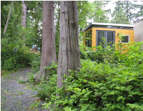
Photo 9.4: Current condition of the main entrance (E1) at the Northwest Stream Center (Hanson 2011)
