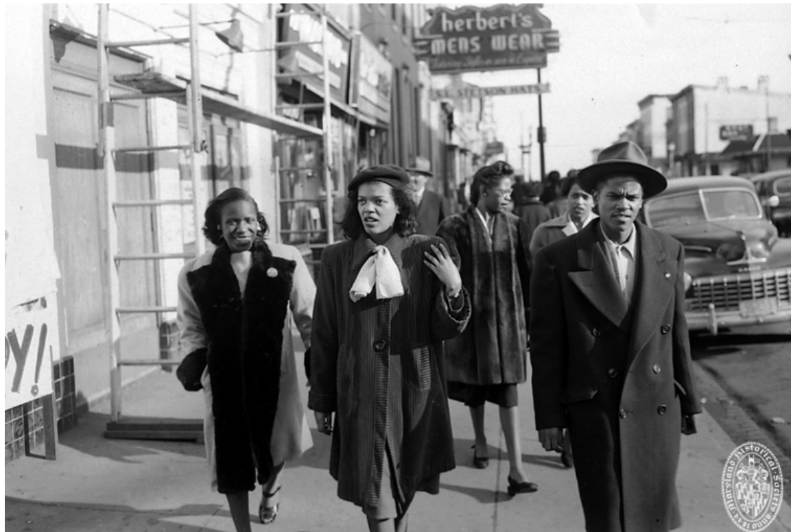
Figure 1.1 Image courtesy of Baltimore Historical Society Pennsylvania Avenue was the place to be during its hayday.
