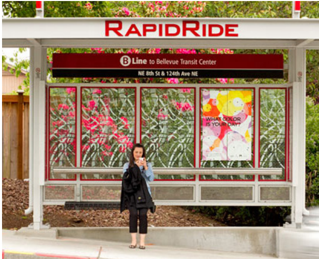
Figure 6.16: King County Metro bus shelter decorated with stained glass art (Source: 4Culture, 2012)
