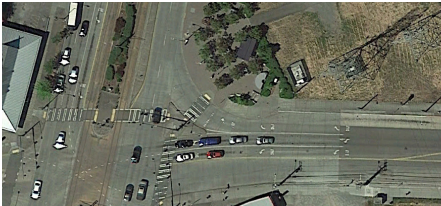
Figure 7.13: An example of a slip lane at the corner of S Henderson St. and Martin Luther King Jr. Way S (Source: Google Earth, 2017)
