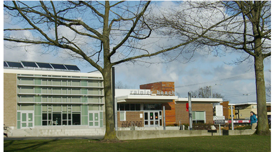
Figure 4.4: South Shore K-8 campus (Source: Seattle Department of Transportation, n.d.)
