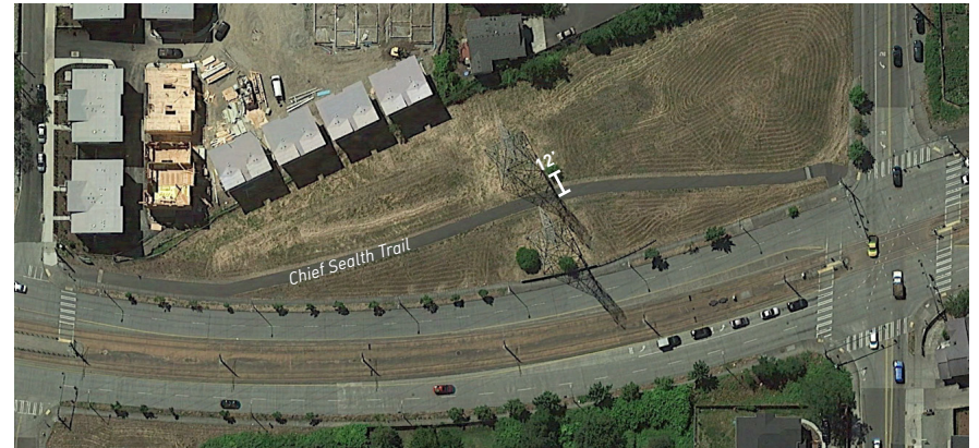
Figure 7.4: A minimum of 12 feet is maintained between Chief Sealth Trail and the transmission towers (Source: Google Earth, 2017)
