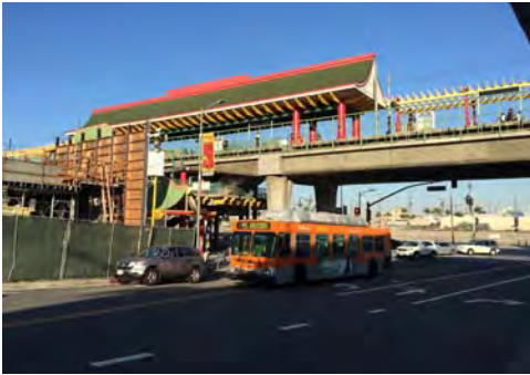
Figure 5.1.22 Metro station in Chinatown
