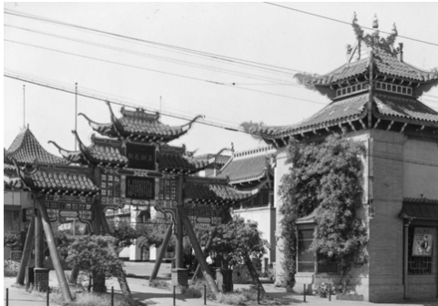
Figure 4.13 New Chinatown opened in 1938 on the site of L.A.’s former Sonoratown
