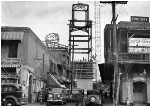
Figure 4.12 LA old Chinatown with the construction of Union Station in the back
