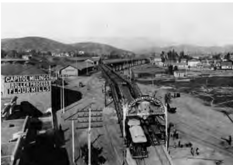
Figure 4.4 Los Angeles Cable Railroad viaduct at Spring Street and College Street, 1888
