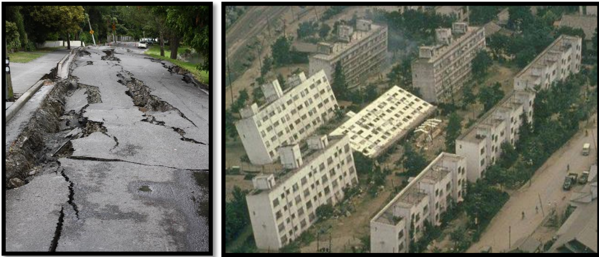
Figure 1: Damage to infrastructure from liquefaction events. (left) River Road, Christchurch New Zealand damaged from lateral spreading in the 2011 earthquake series. (right) A dramatic example of sinking apartment buildings due to the loss of soil shear strength, Nigata, Japan 1964.
