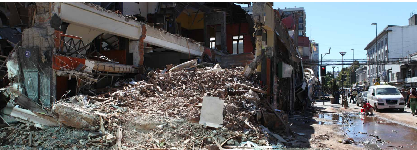
▲ Damage to structures in downtown Concepcion, Chile, due to the February 27, 2010, magnitude 8.8 earthquake.
