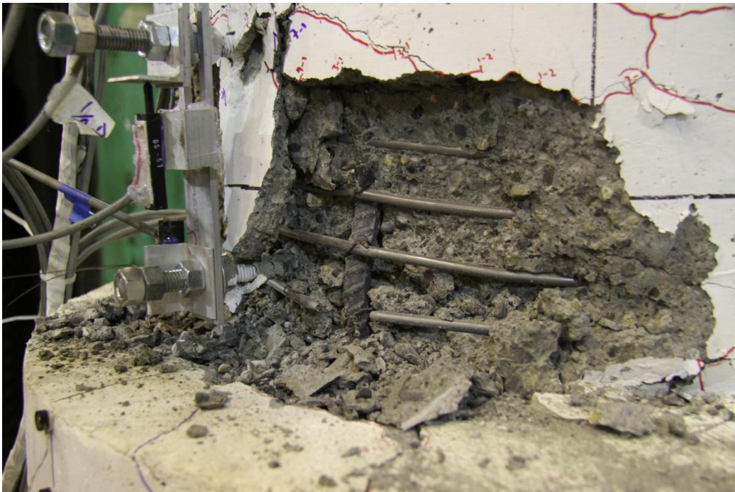
Figure C-0-5. DS-1 – First column spiral fractured in Cycle 10-1 (8.43/-8.27 percent drift)
