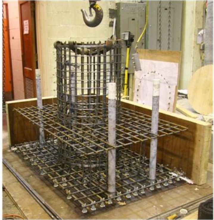
b). Shaft-Footing reinforcement
