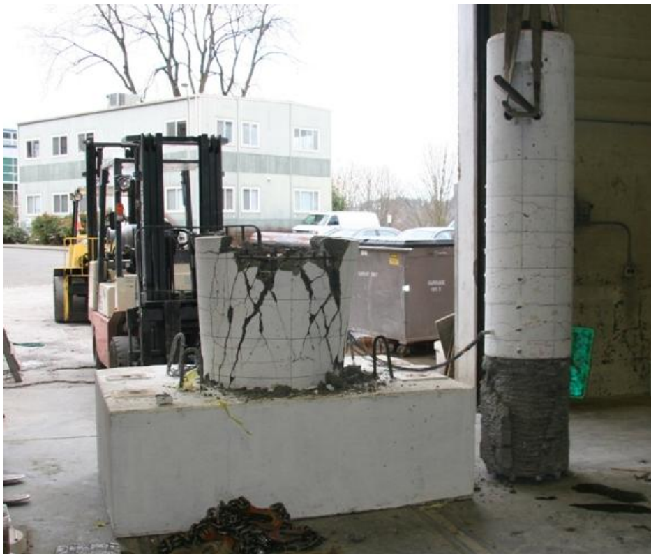
Figure 4-3. Specimen DS-2 after testing
