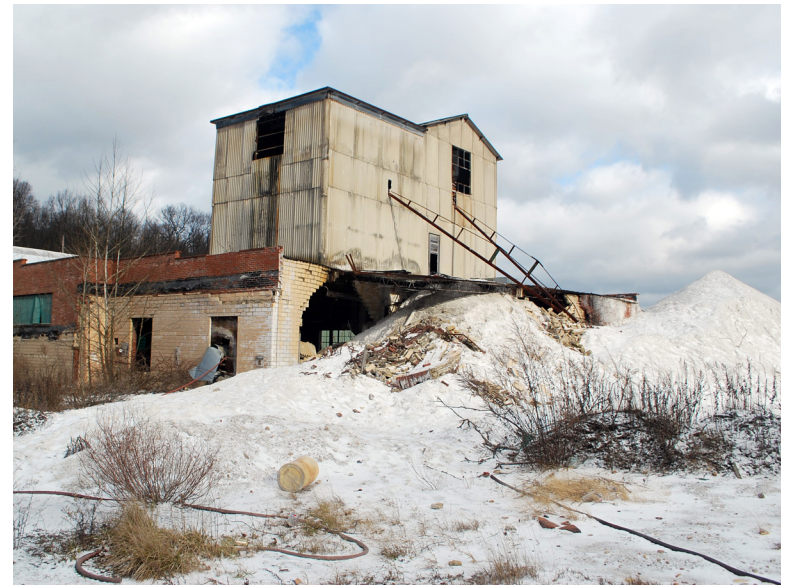
Abandoned brick factory in my hometown, South Beaver Twp, PA. [Leann Andrews]
