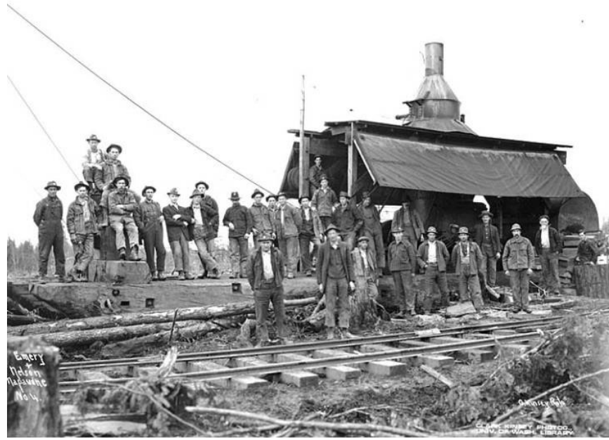
Figure 2.5 Timber workers on a steam donkey. Source: Clark Kinsey. https://digitalcollections.lib.washington.edu/digital/collection/clarkkinsey/id/214/rec/7 .
