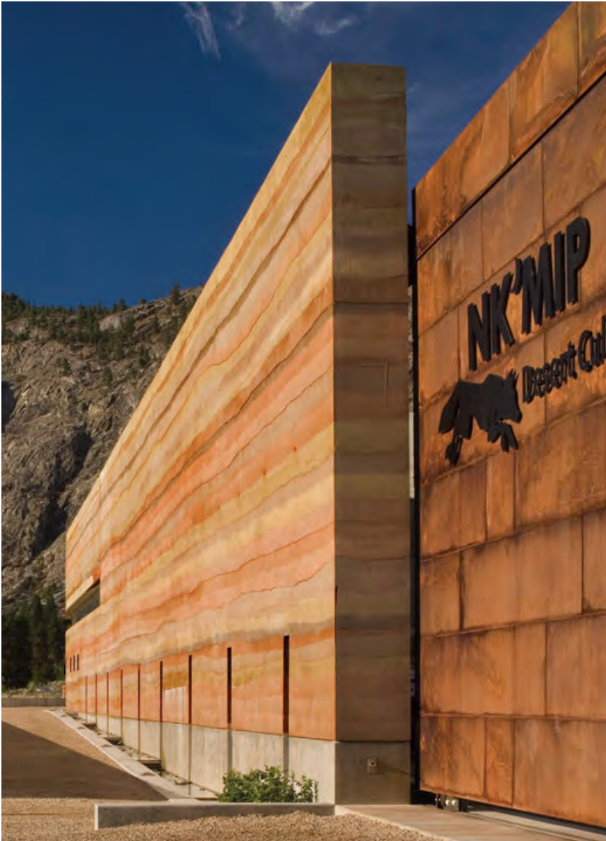
figure 39: Nk'Mip Desert Cultural Center rammed earth wall | Osoyoos, BC
