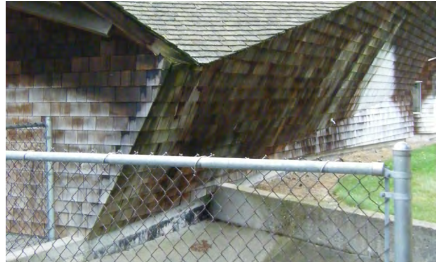
figure 30: Seabird Island School fencing
