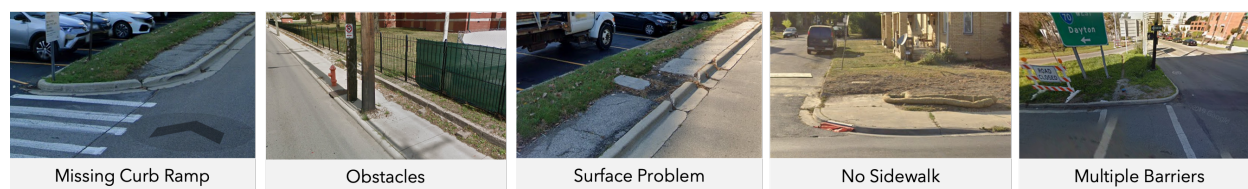
Figure 3.1: Examples of sidewalk accessibility barriers. The last sub-figure shows multiple barriers present together: missing ramp, no sidewalk, and uneven surface.
