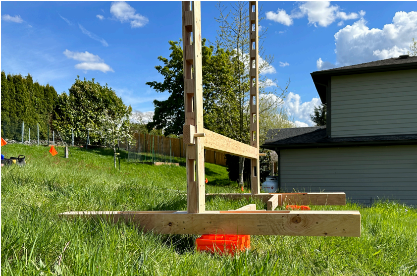
Fig. 85 FFS requires each base to be individually leveled
