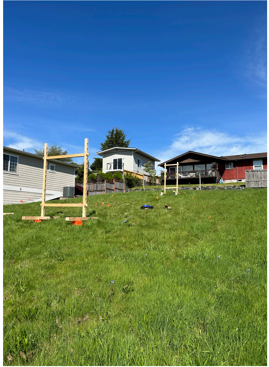
Fig. 75 Using two frames to test elevations
