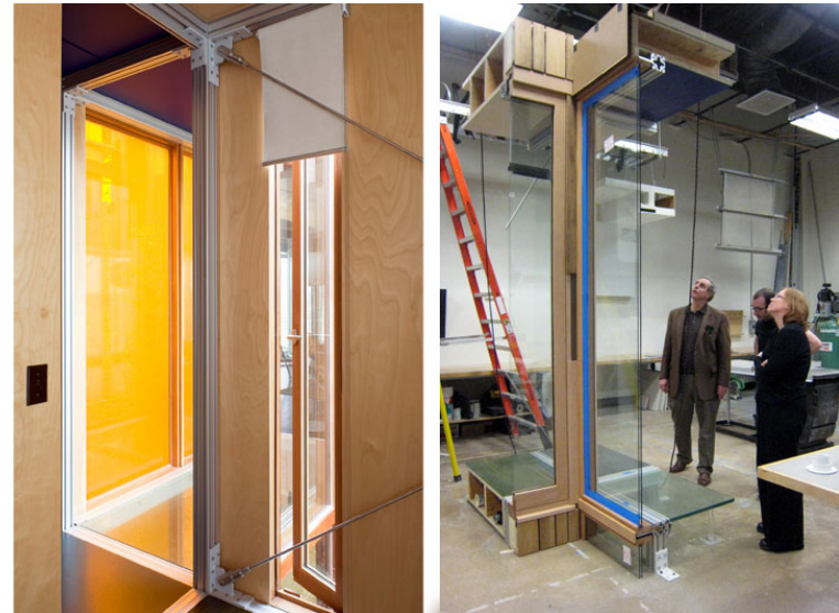
Fig. 5 Full-scale mock ups of a built detail (left) and reconstructed detail (right), KieranTimberlake
