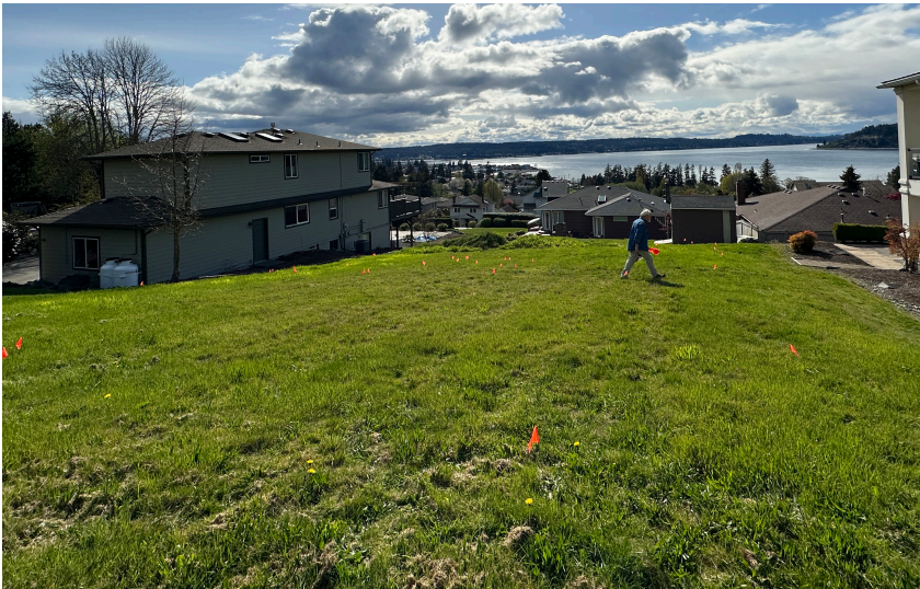
Fig. 59 Laying out the core patterns on site with orange flags
