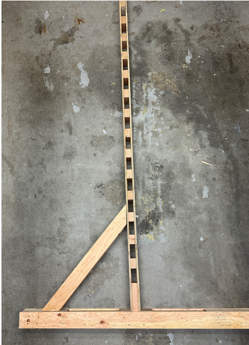
Fig. 67 Upright & lateral bracing attached to base assembly for FFS
