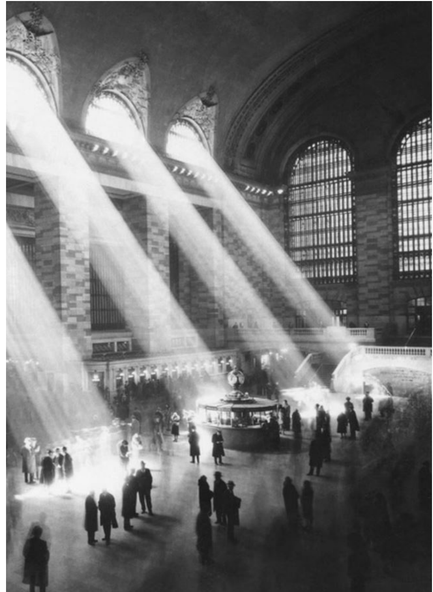
Fig. 13 Clerestory Light in Grand Central Station, NY
