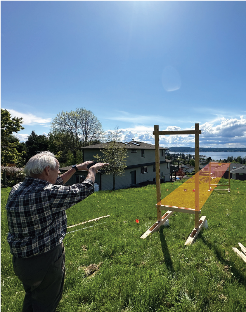
Fig. 71 Finding the elevation of the main entrance floor plate
