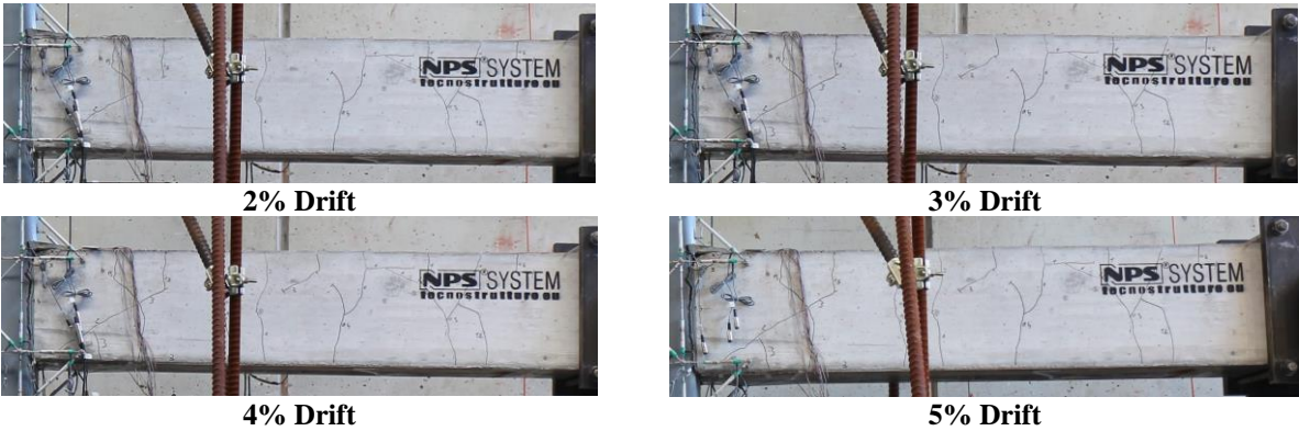
Figure 5.40: NPS4e - Beam Cracking Propagation
