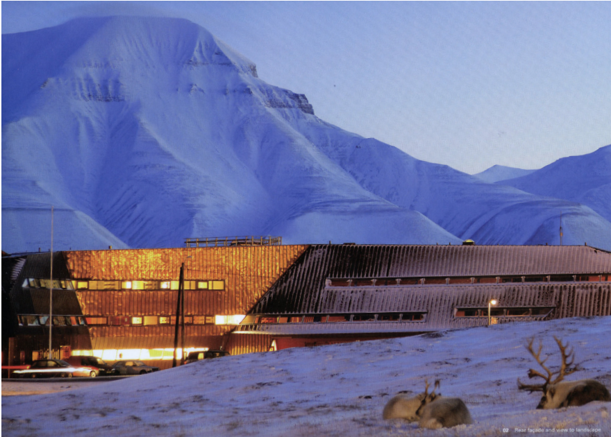
Figure - 34 Exterior view of the center during winter
