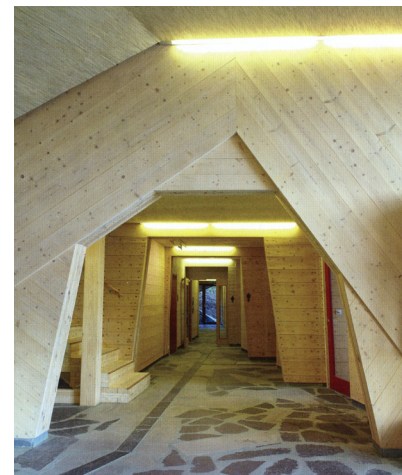
Figure - 43 Hallway showing Holz100
