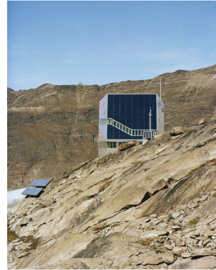
Figure - 21 South Facade with PV Panels
