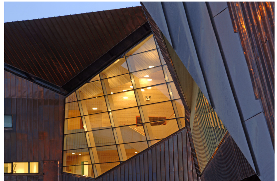
Figure - 31 Exterior view showing zinc cladding
