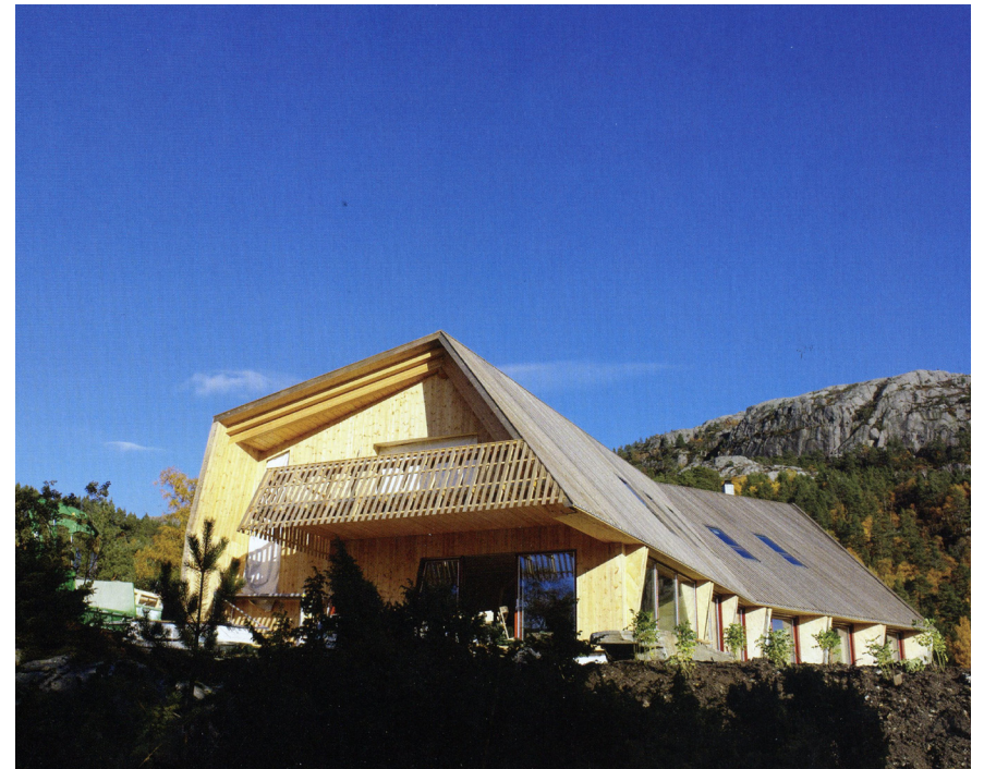
Figure - 40 Exterior view
