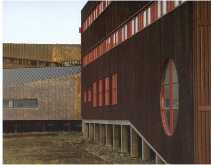
Figure - 33 Exterior view showing the raised foundation
