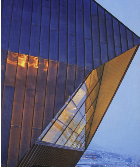
Figure - 32 Exterior view
