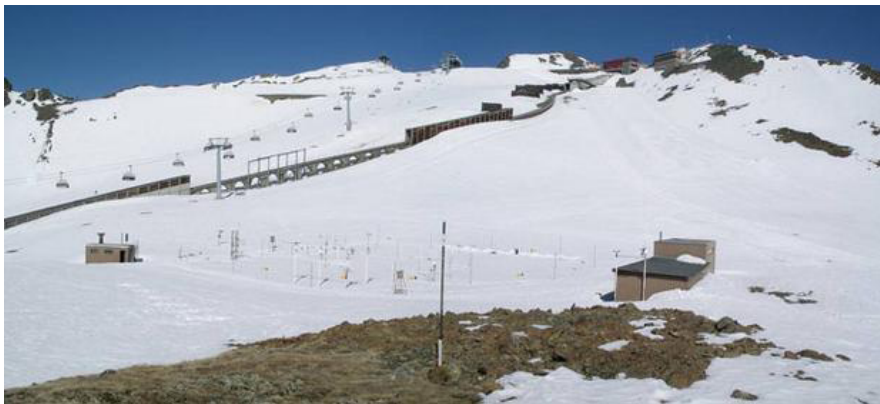
Figure - 45 Exterior view of shed and research equipment
