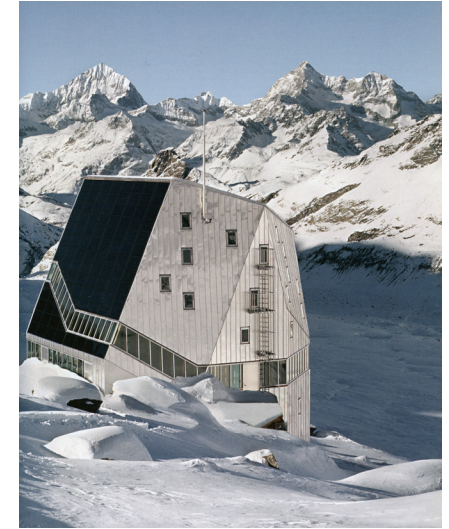
Figure - 22 Exterior View
