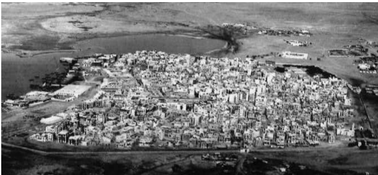
Fig 7. 1938 Aerial view of the Old City of Jeddah by Wikipedia . Retrieved Nov 05
