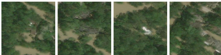
Figure 1.2: Flooded/Damaged samples cropped from the original imagery.
