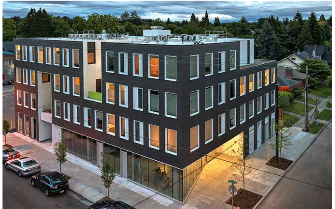
Fig. 3.7 Photograph of 3360 SE Division
