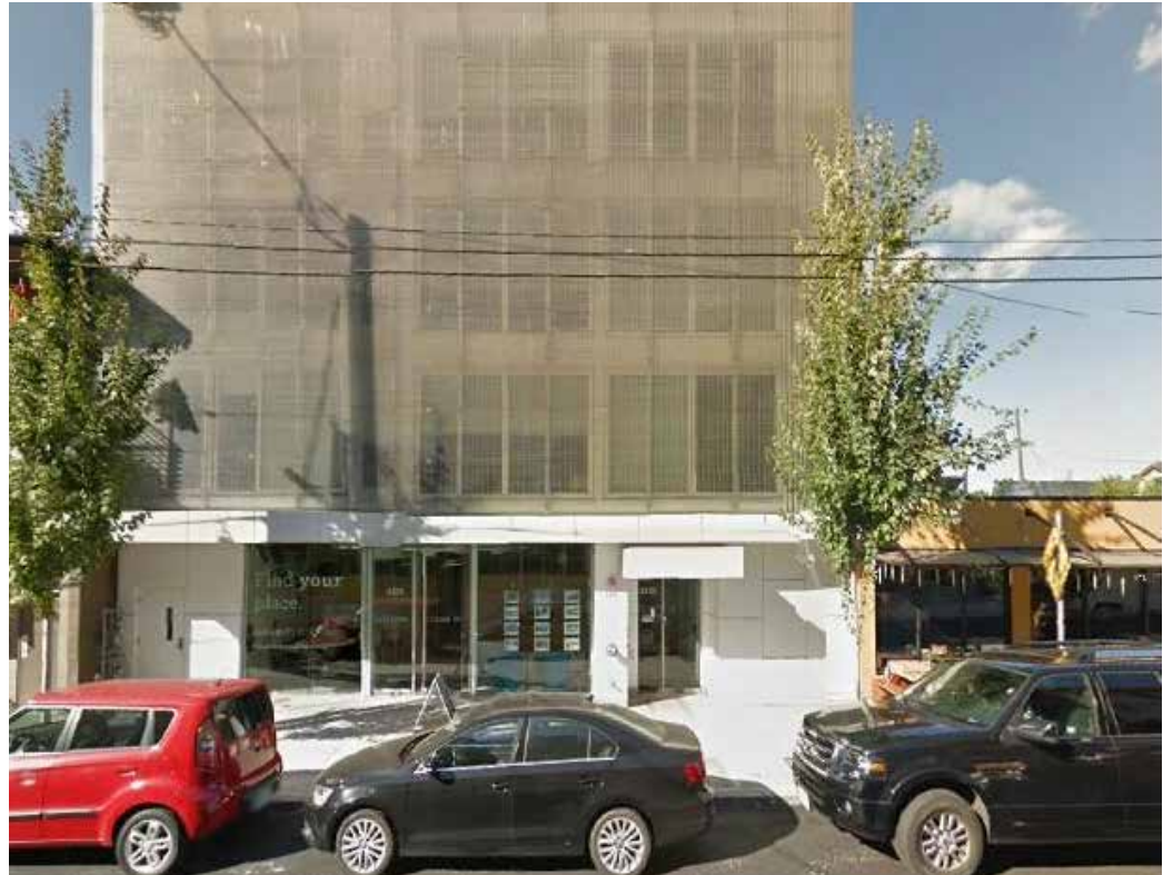
Fig. 3.11 Photograph of 3125 SE Division
