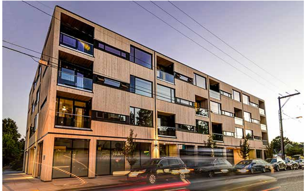
Fig. 3.9 Photograph of 3330 SE Division
