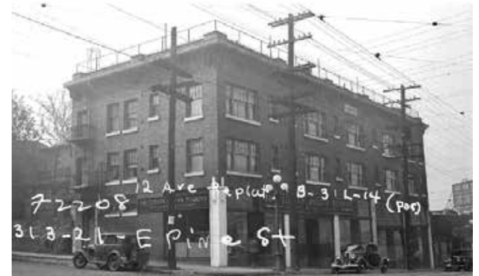
Fig. 2.33 Timkin Roller Bearing Building, ca. 1937
