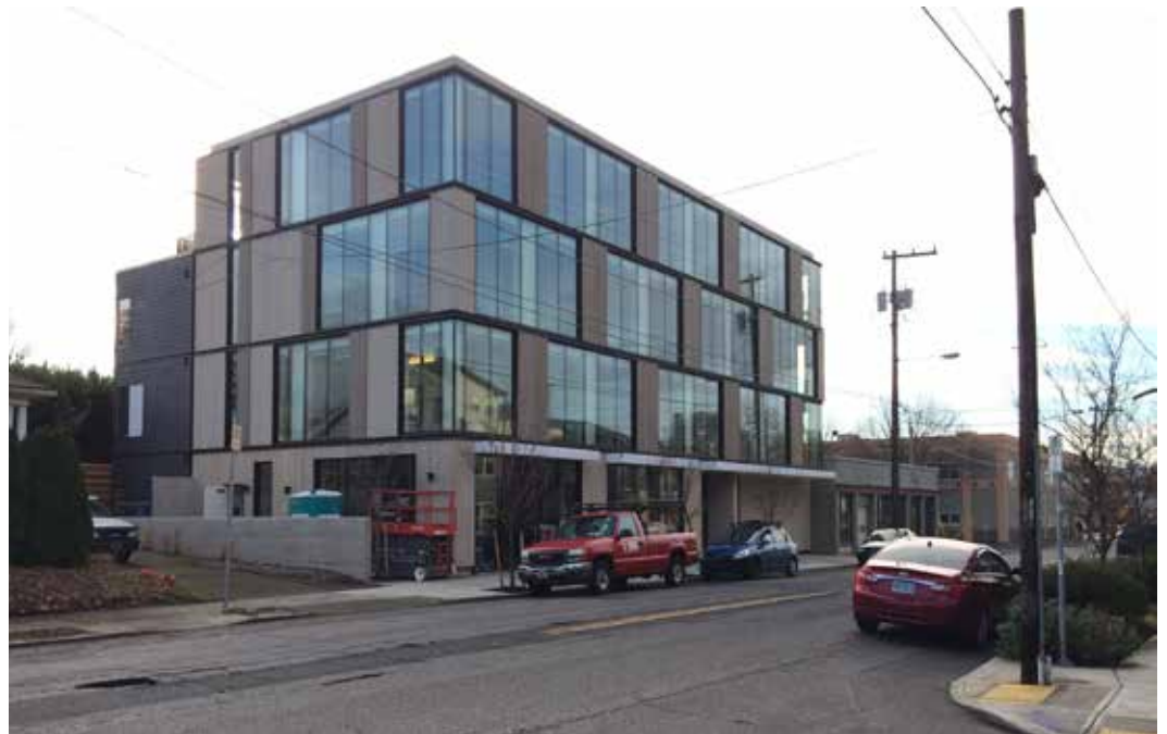
Fig. 3.15 Photograph of 4330 SE Division
