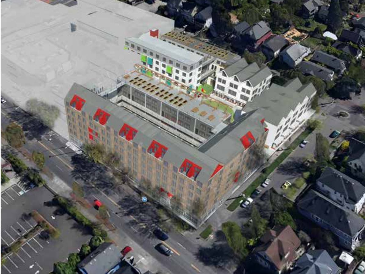
Fig. 4.49 Site A: birdseye view. Incisions into the mass provide balconies and introduce color and depth to the otherwise flat elevations.
