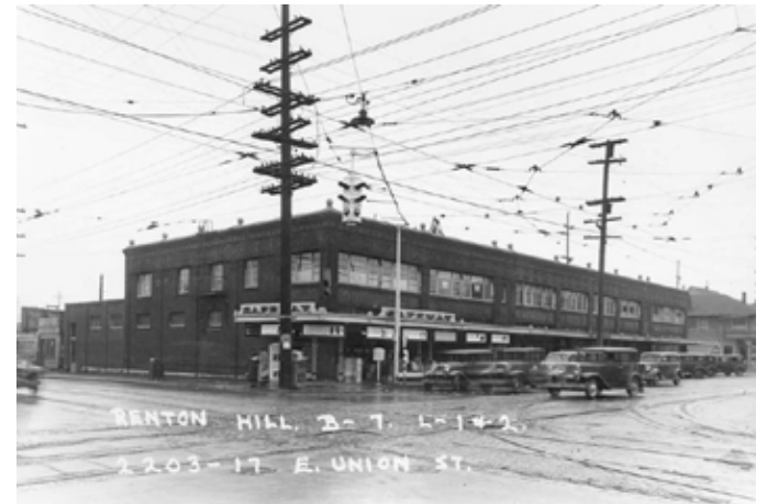
Fig. 4.4 23rd and Union St. ca. 1937, view facing southwest. Streetcar tracks occupied both rights-of-way.
