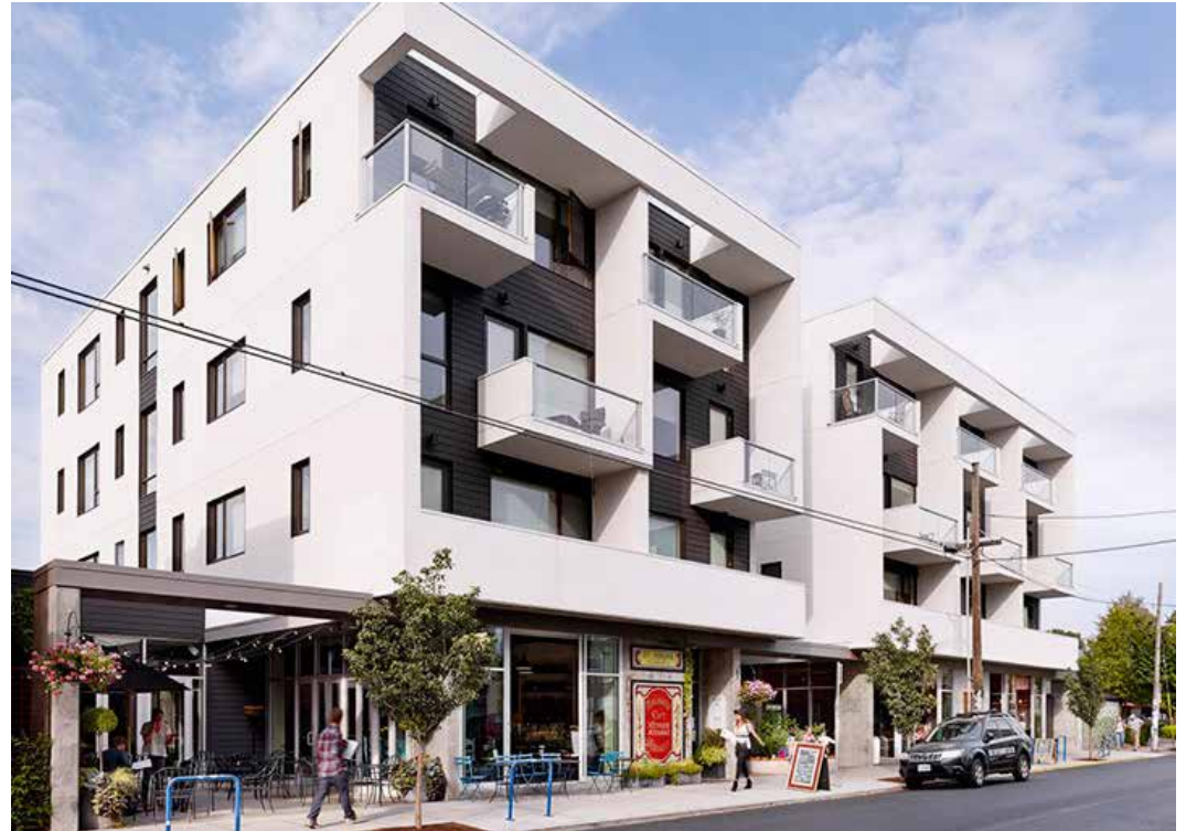
Fig. 3.5 Photograph of 3339 SE Division
