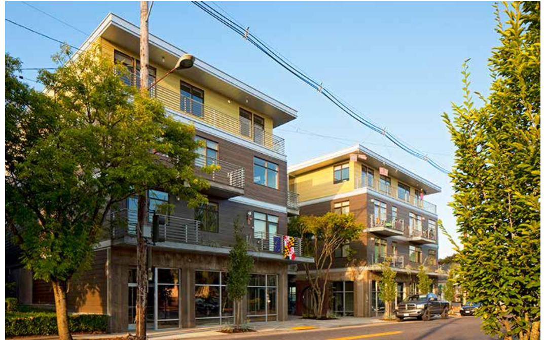
Fig. 3.13 Photograph of 3810 SE Division
