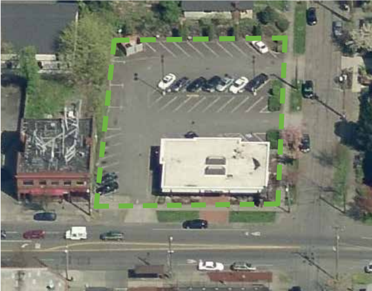
Fig. 4.28 Site of proposed Capitol Hill Housing development at 24th Union.
