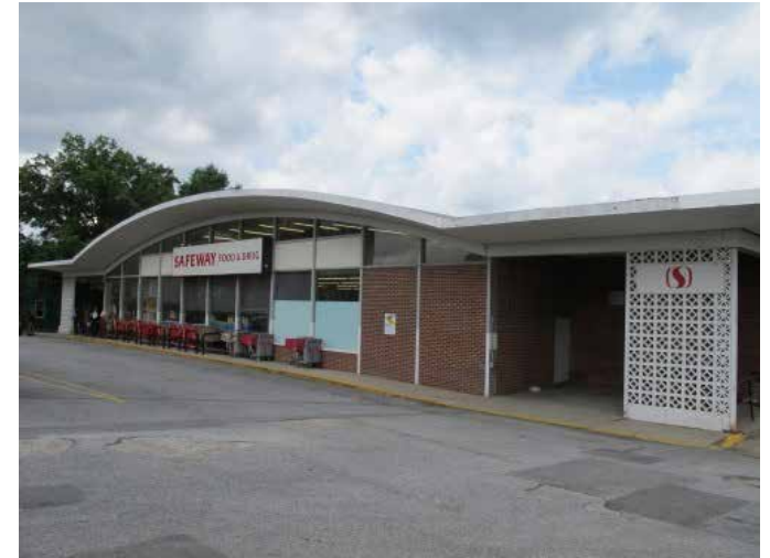
Fig. 2.59 Standardized suburban type Safeway store, constructed ca. 1965
