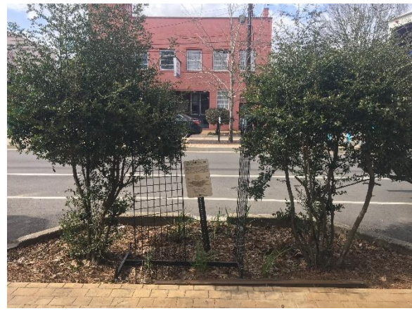
Figure V-C Bioswale Curb Extension on O.C. Haley
