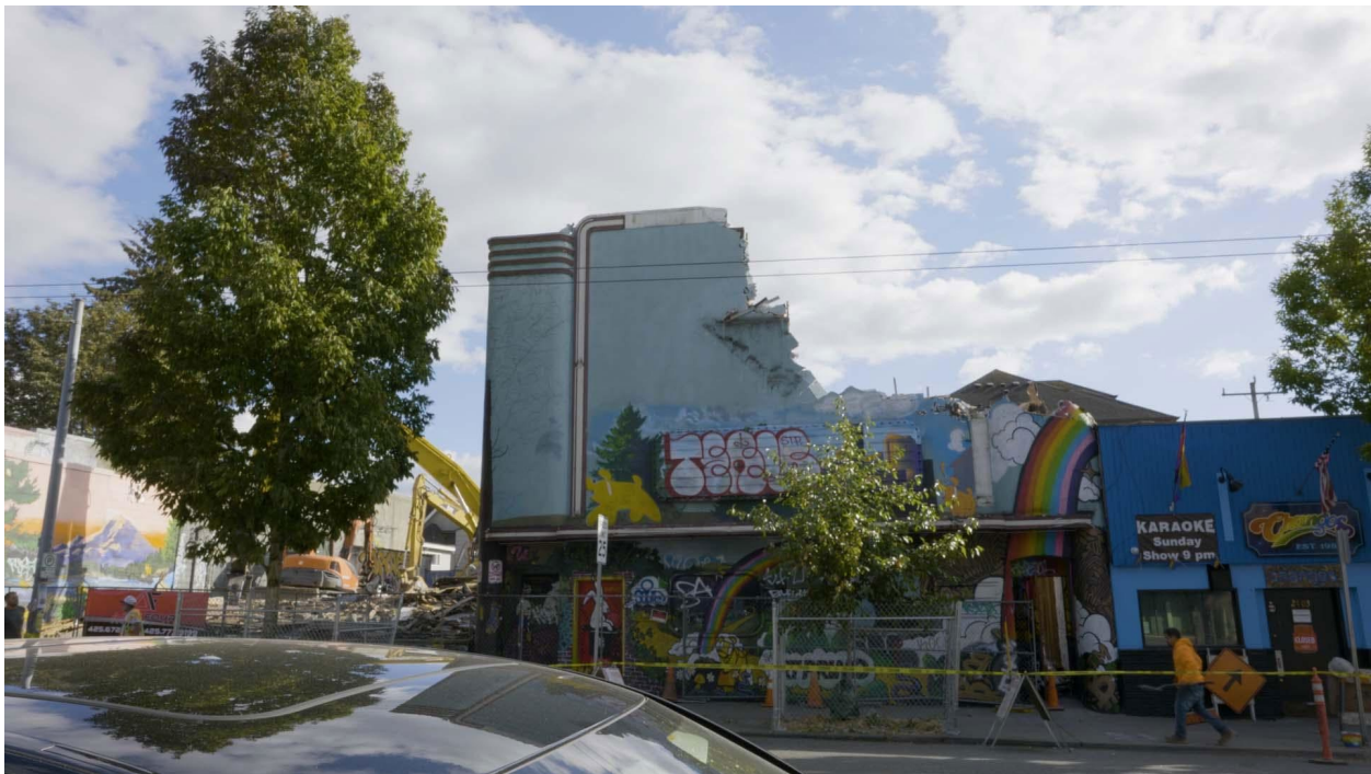
Figure 6.7 The Guild as it gets demolished (19 min, 57 sec)
