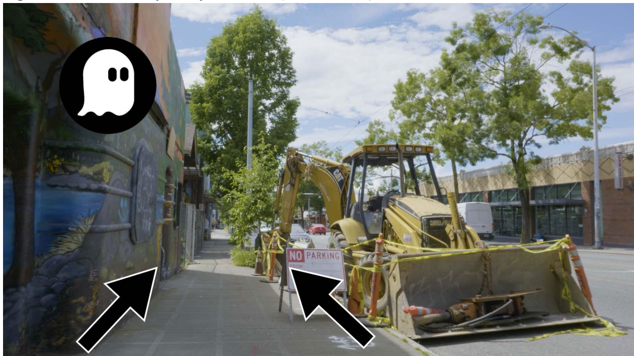
Figure 6.2 Bulldozer in front of The Guild (6 min, 50 sec)
