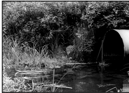
A culvert in Stossel Creek
