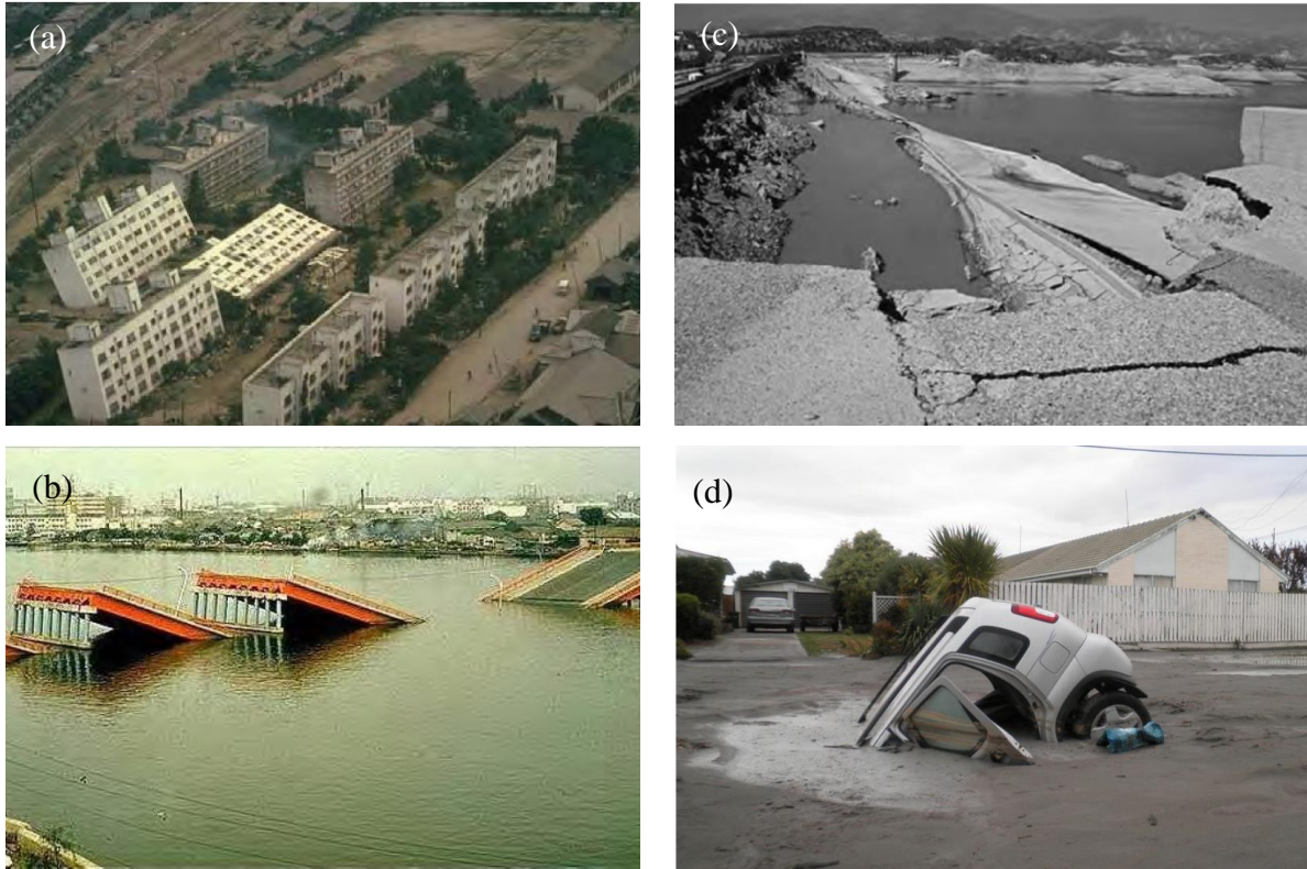
Figure 2.1: Photos of damage due to liquefaction. (a) Foundation failure of the Kawagishi-Cho apartments from the 1964 Niigata earthquake (from National Information Service for Earthquake Engineering, 2016). (b) Lateral spreading failure of the Showa Bridge from the 1964 Niigata earthquake (from National Information Service for Earthquake Engineering, 2016). (c) Crest failure of the Lower San Fernando Dam after the 1971 San Fernando earthquake (from National Information Service for Earthquake Engineering, 2016). (d) Large sand boil in Christchurch from the 2011 Christchurch earthquake (from Cubrinovski et al., 2011).
