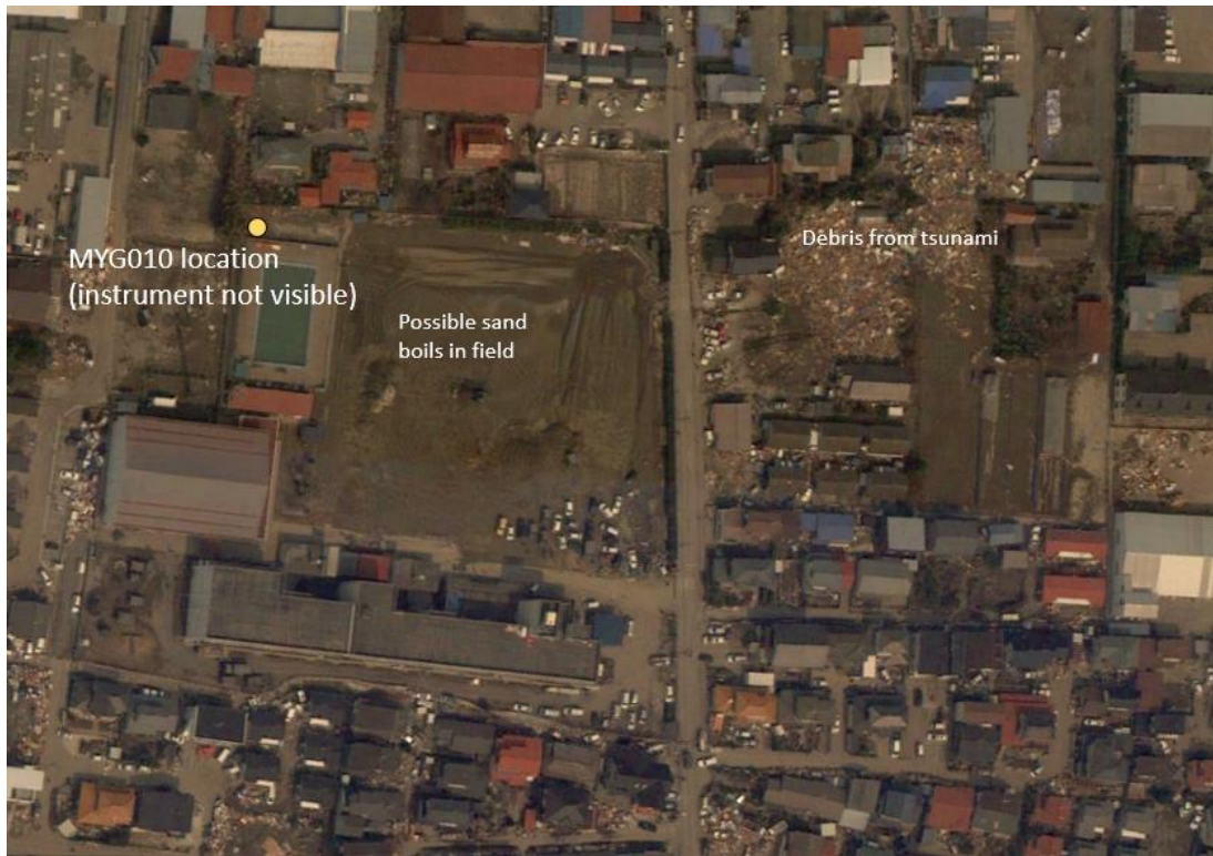
Figure 7.32: Aerial photo showing debris and damage at MYG010 after Tohoku earthquake. Aerial photo of the site taken on March 28, 2011. Image courtesy of Google Earth.
