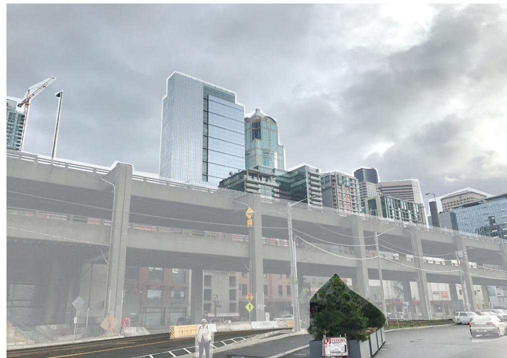
fig. 85 - Waterfront Park fig. 86 - Alaskan Way looking east
