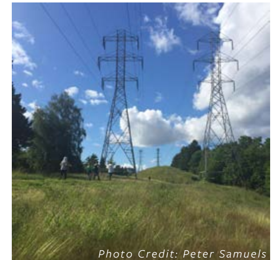
Above: Conservation mowing results on the Chief Sealth Trail
