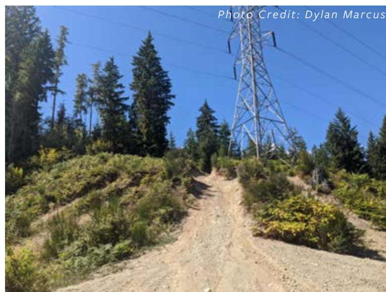
Top Left: Erosion by the transmission tower footings above Rinker Creek resulting from excessive ORV use
