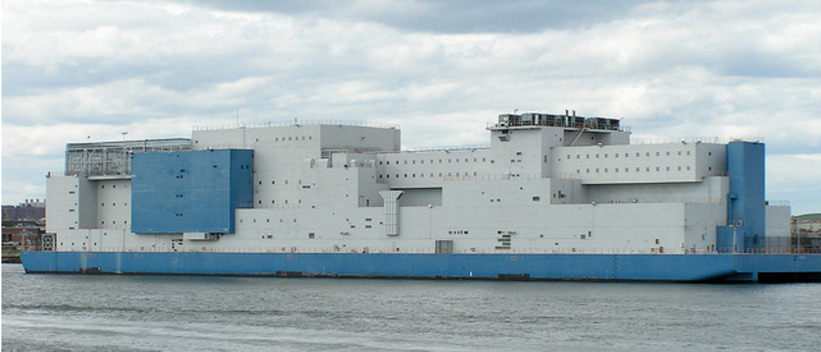
Figure 8: Vernon C. Bain Correctional Facility. Photography courtesy of Reivax New York Press
