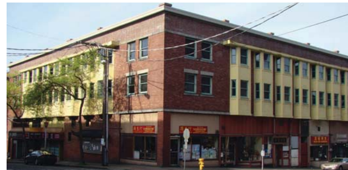
Figure 18. Louisa Hotel, 7th Ave S and S King St
