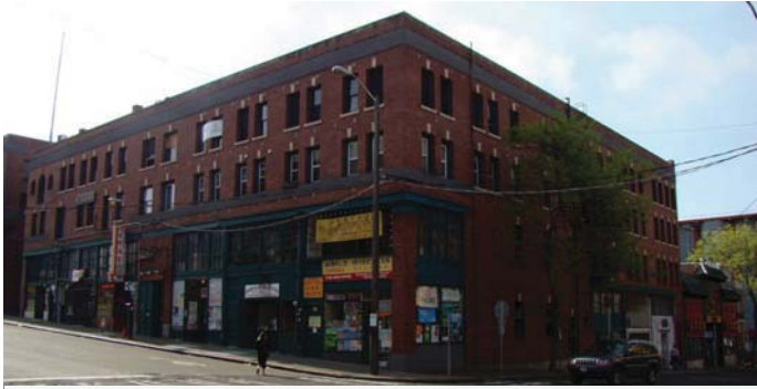
Figure 19. Kong Yick Buildings 7th and King. Author Photo, May 2012.
