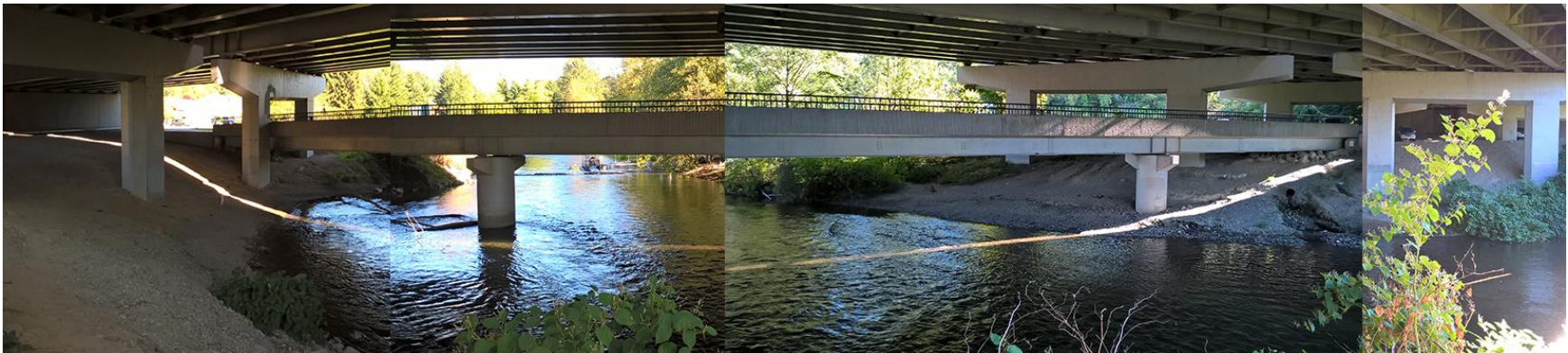
Figure 65 Pedestrian bridge under I-405
